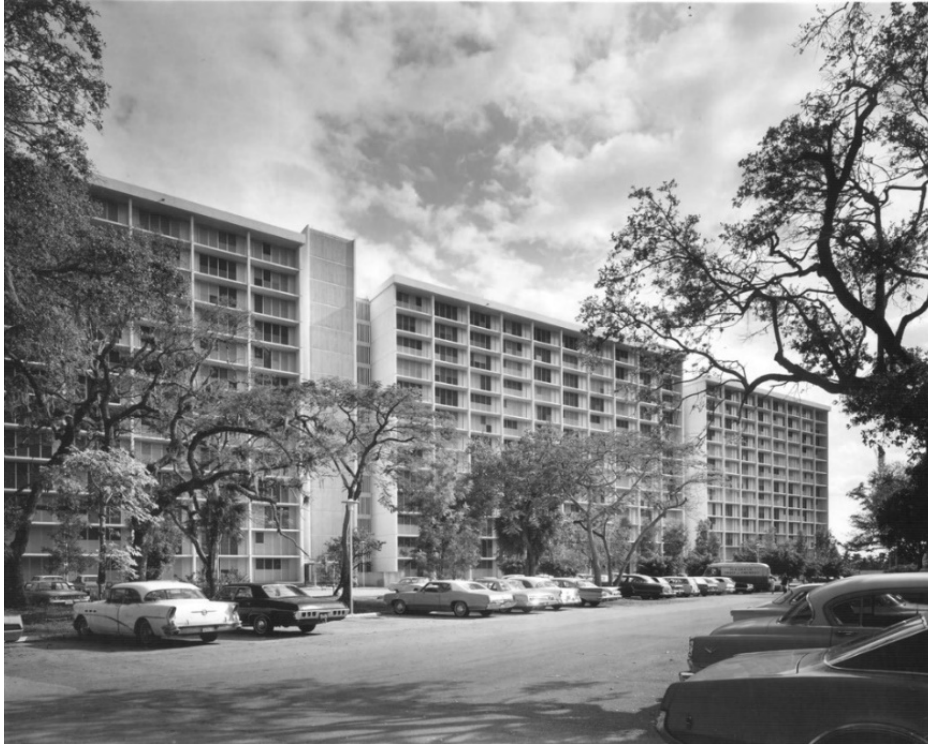
Robert King High Towers, Miami, Ferendino, Grafton, Pancoast, 1964. Photo by Joseph W. Molitor Photography. Courtesy of Spillis Candela DMJM Archive.
