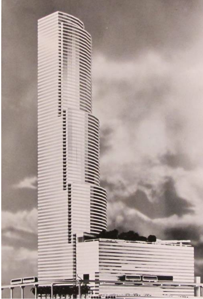
Centrust Tower, Downtown. I.M. Pei + Associates, 1987. SE Second St + First Ave. Designed by I.M. Pei + Associates. May 2, 1985. Courtesy of HistoryMiami Museum, Miami News Collection (1995-277-2065).
