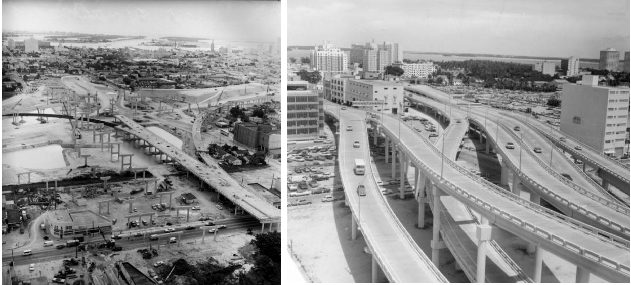
(left) Midtown Expressway Interchange under construction in Overtown. Completed in the mid-1960s. Courtesy of Miami Herald. (right) Express Highway, Miami. Photograph Karl E. Holland, 1969. Florida Memory Department of Commerce Collection (c673686)
