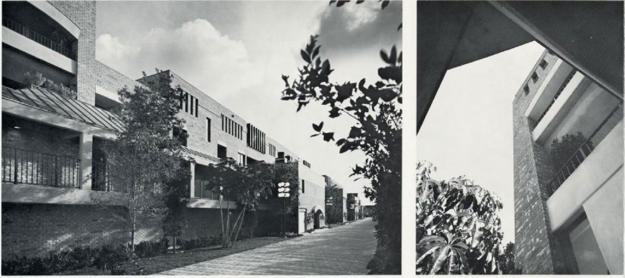
Townhouses at Quayside, North Miami. Alfred Browning Parker, 1974. Courtesy of George A. Smathers Libraries, University of Florida, Alfred Browning Parker Collection.
