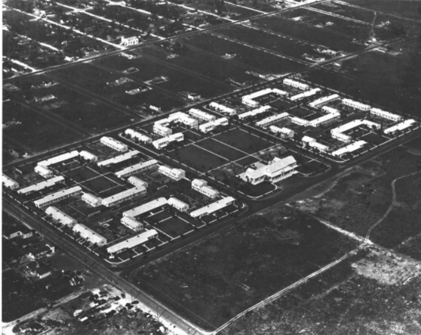
Liberty Square, Liberty City, Miami, Paist and Stewart with associate architects Robert Law Weed, Vladimir Virrick and E.L. Robertson, 1934-37. From Raymond Mohl, "Shadows in the Sunshine: Race and Ethnicity in Miami," Tequesta, January 1989. p. 70.
