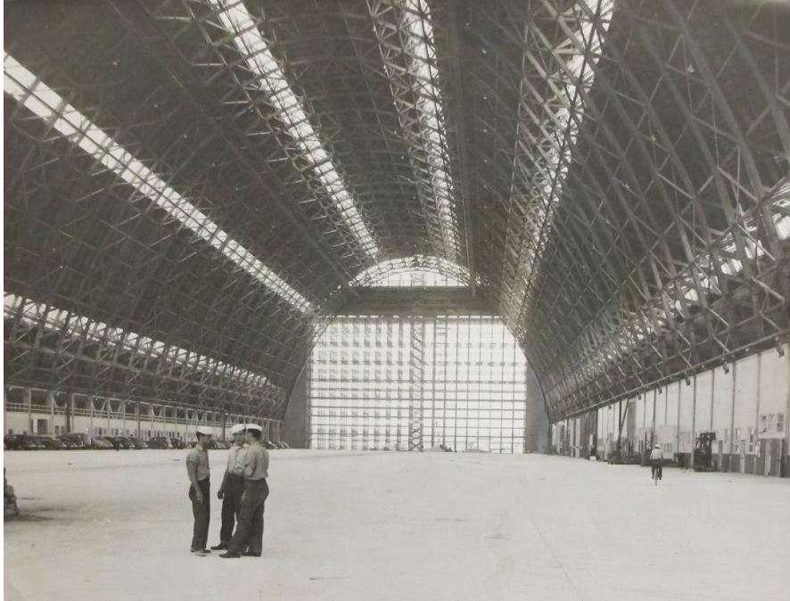
Blimp Hangar at Richmond Naval Air Station, c. 1943. Photographer unknown. Courtesy of HistoryMiami Museum, Miami News Collection.
