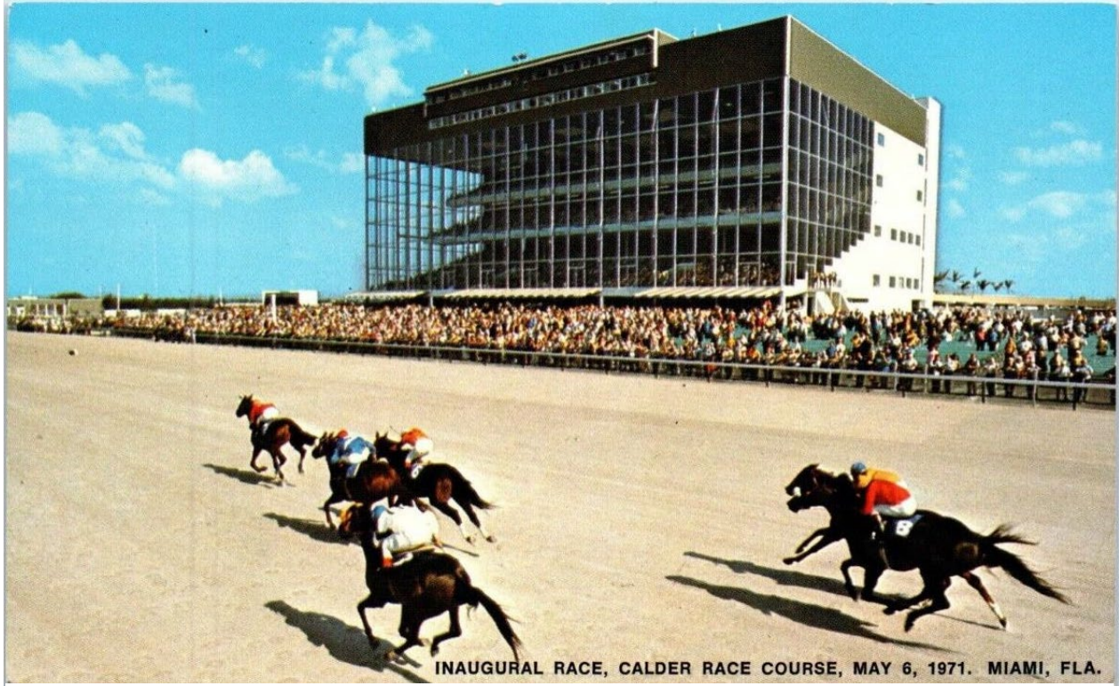
Calder Race Track, Dade County, Stefan Zachar, 1971. Demolished. Unidentified postcard of inaugural race, c. 1972.
