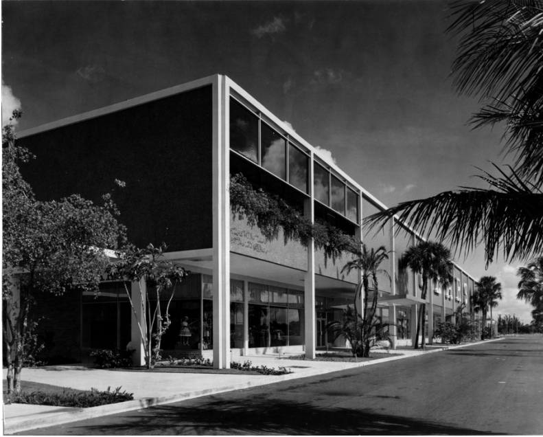
Northside Shopping Center, Dade County. View of corner. Weed & Johnson Associates, 1960. Photograph by DuPont Plaza Photography. Courtesy of Johnson Associates Architects, Inc.
