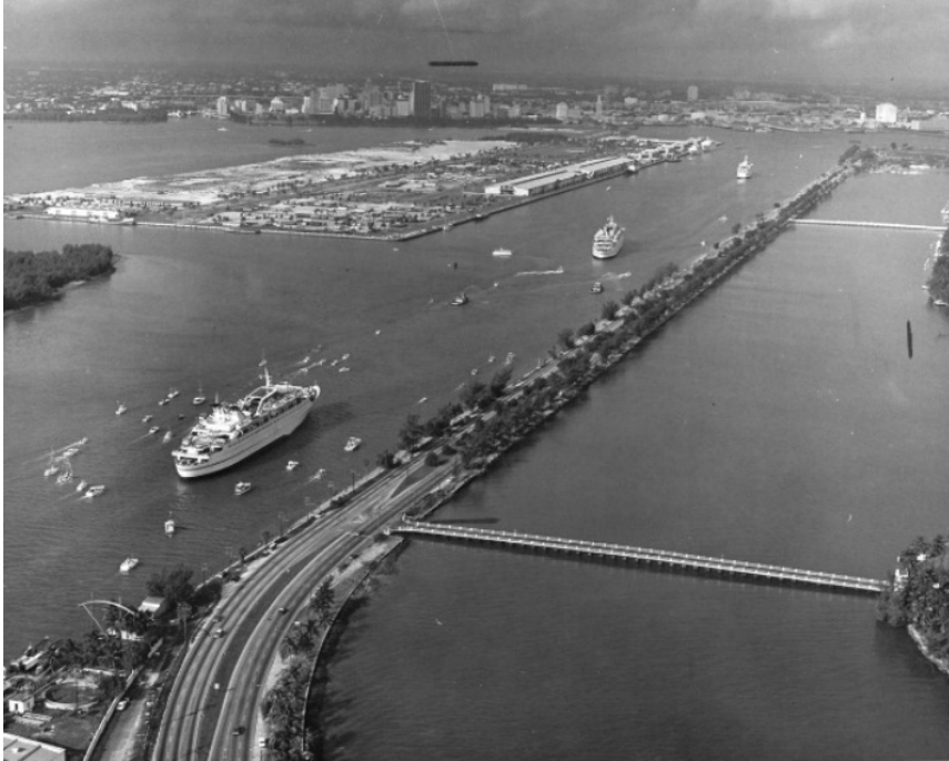
Construction of new port on Dodge Island, Miami. Photo by Martine Aronow. Courtesy of HistoryMiami Museum, Miami News Collection.
