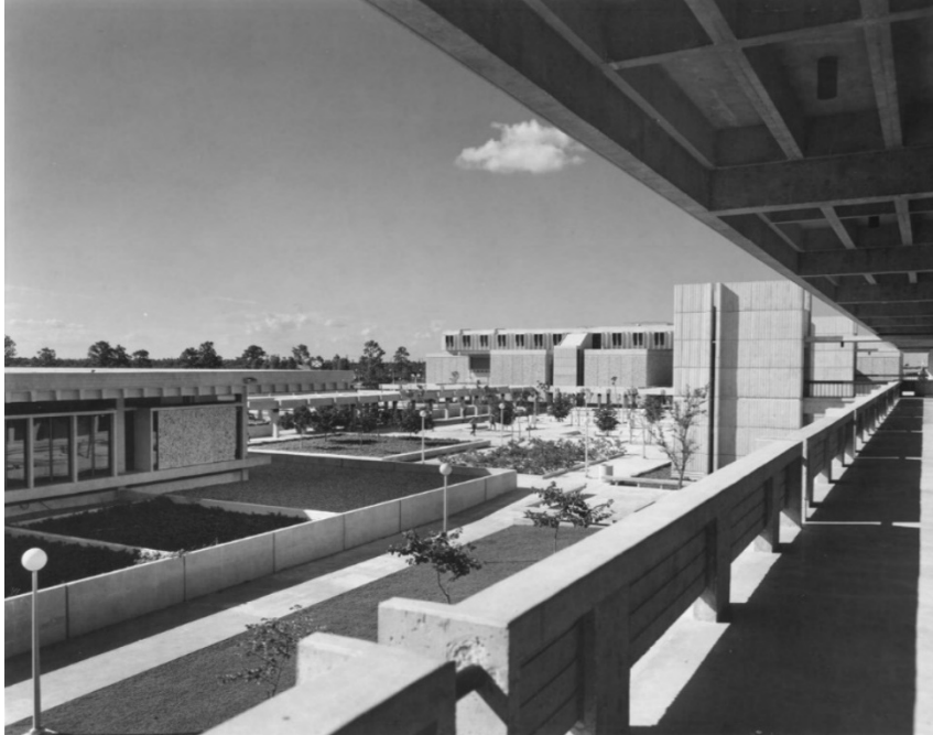
Administration Building and Science Building, Miami-Dade Junior College, South Campus, Kendall. Pancoast, Ferendino, Grafton, 1967. Photo by Joseph W. Molitor Photography. Courtesy of Spillis Candela DMJM Archive.
