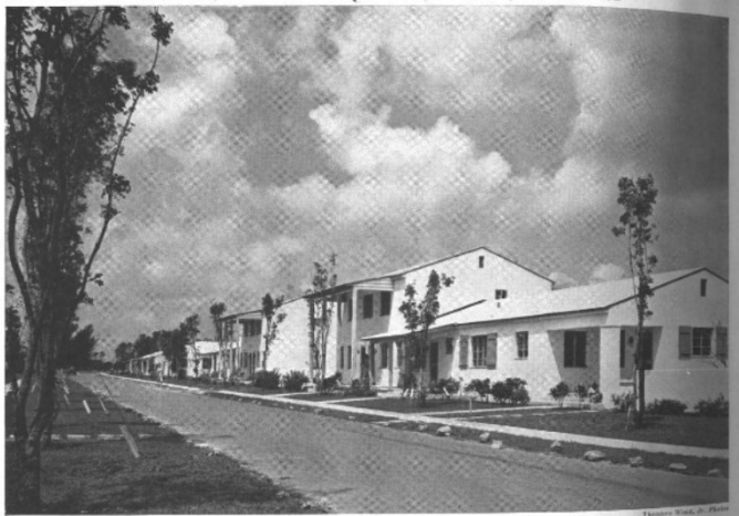
Liberty Square public housing project, Miami. Phineas E. Paist, C. Sheldon Tucker, Harold Steward, Walter C. De Garmo, E. L. Robertson and V. E. Virrick architects, 1937. Courtesy of HistoryMiami Museum.
