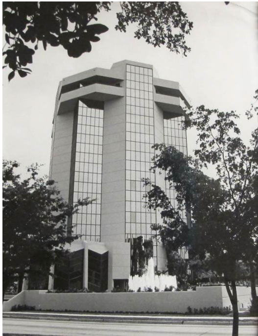
Citizens Federal Savings & Loan, Miami. Morris Lapidus, 1975. Photo by Ray Fisher, 1975. Courtesy of HistoryMiami Museum, Miami News Collection (1995-277-2581).
