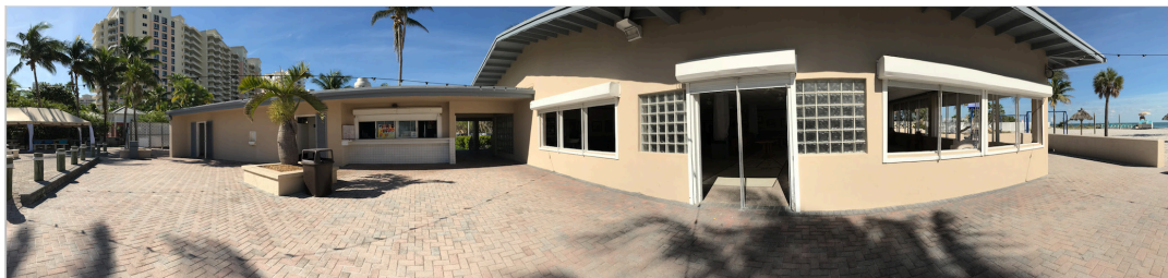
Panorama taken towards West, closer to the structure (2017).
