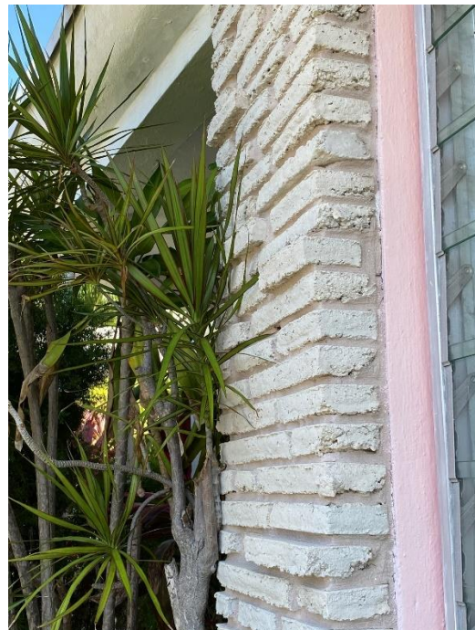
Façade detailing showing the exterior brick. The brick is not a veneer, but full bricks arranged in a staggered pattern with bricks projecting at various depths.
