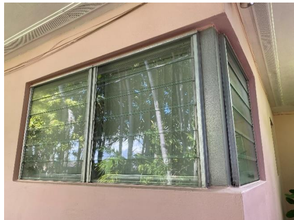
Corner jalousie windows on the west elevation.
