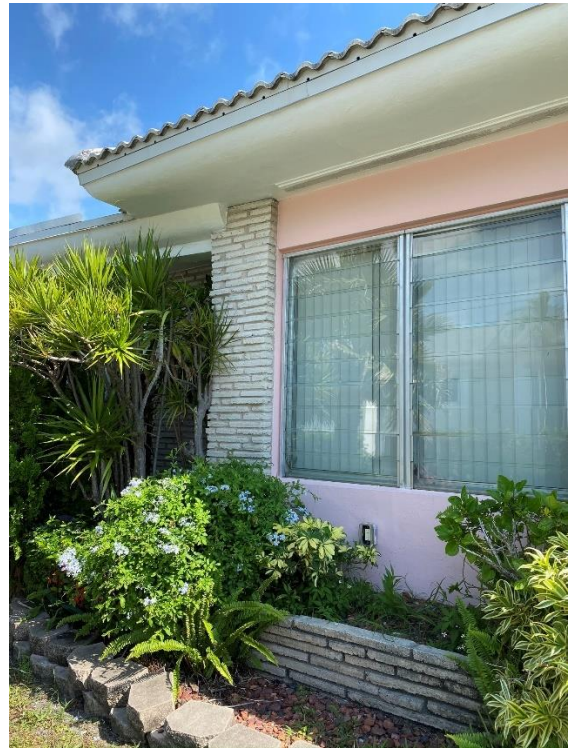
Façade of Fisher-Sapero Residence illustrating unique architectural features: wide eaves, barrel tile roof, jalousie windows, brick and stucco exterior, and integrated planters.
