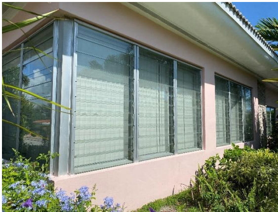
East elevation showing original jalousie windows with corner wrapping.
