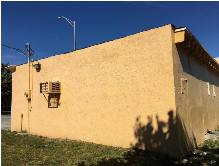
South elevation of c.1958 addition with portion of rear/east elevation illustrated at right.
