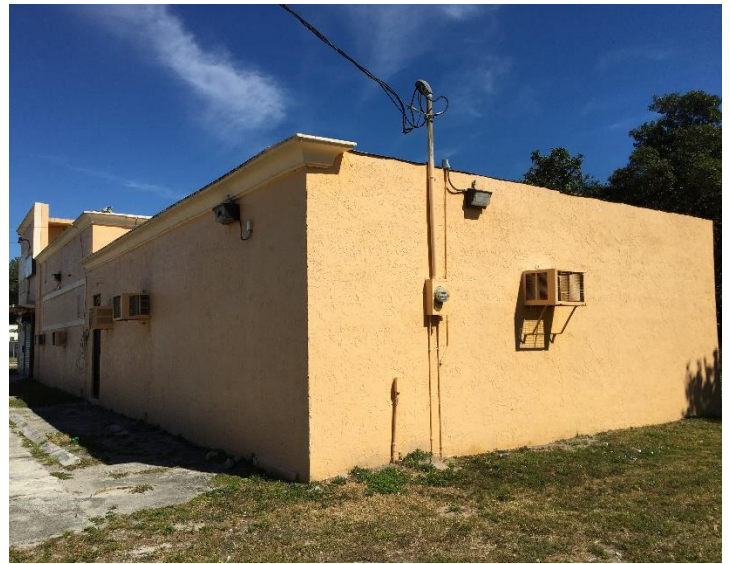
Southwest corner of c.1958 addition showing south elevation and showing façade of what was the c.1958 addition.
