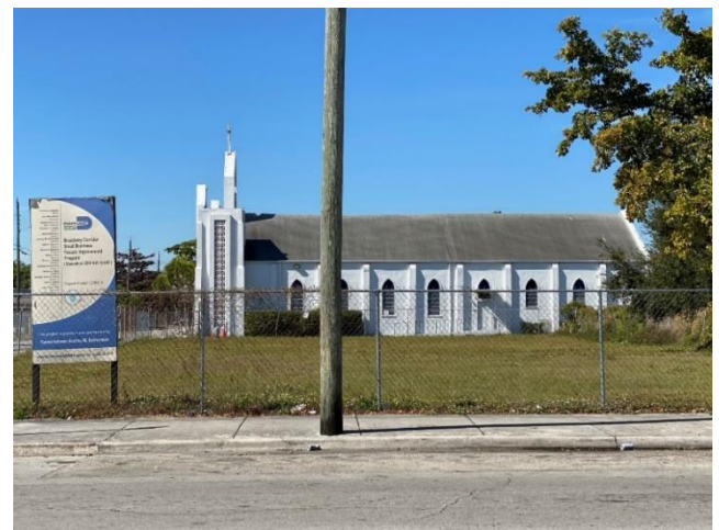
St. James AME Church to the west of the Liberty Lodge, visible across vacant property.
