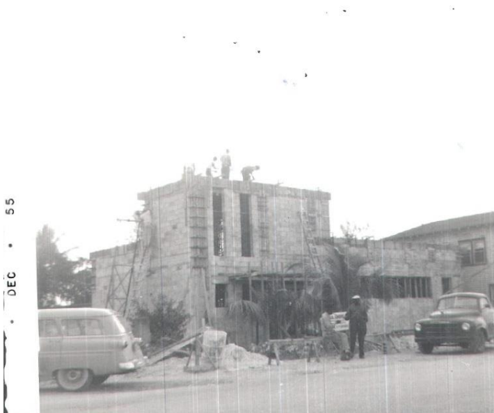
Lodge under construction, Dec. 1955. The two-story building is seen at right on the lot that would soon house the c.1958 addition.
