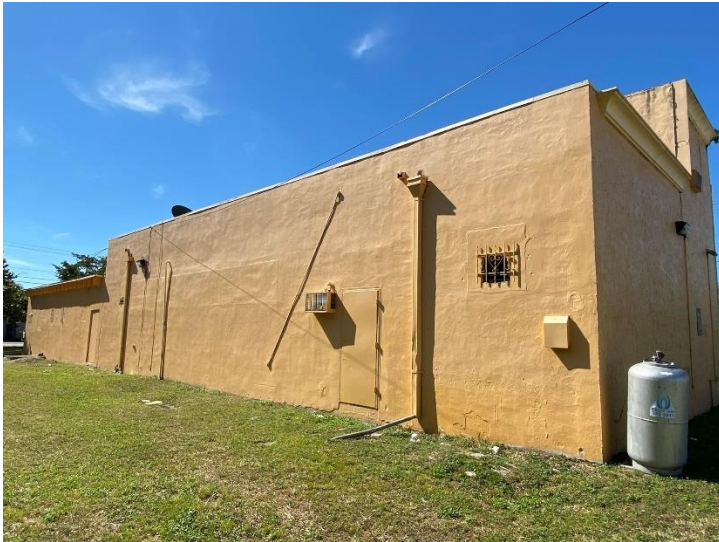
Rear/east elevation showing c.1956 structure.
