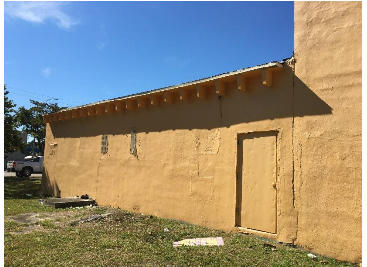
Rear/east elevation showing c.1958 addition, since altered from original construction that included windows and two exterior doors.
