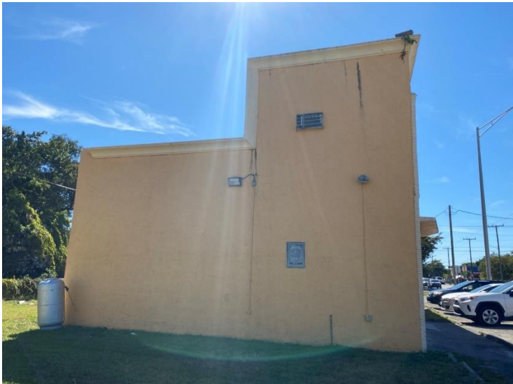
North elevation of c.1956 structure.
