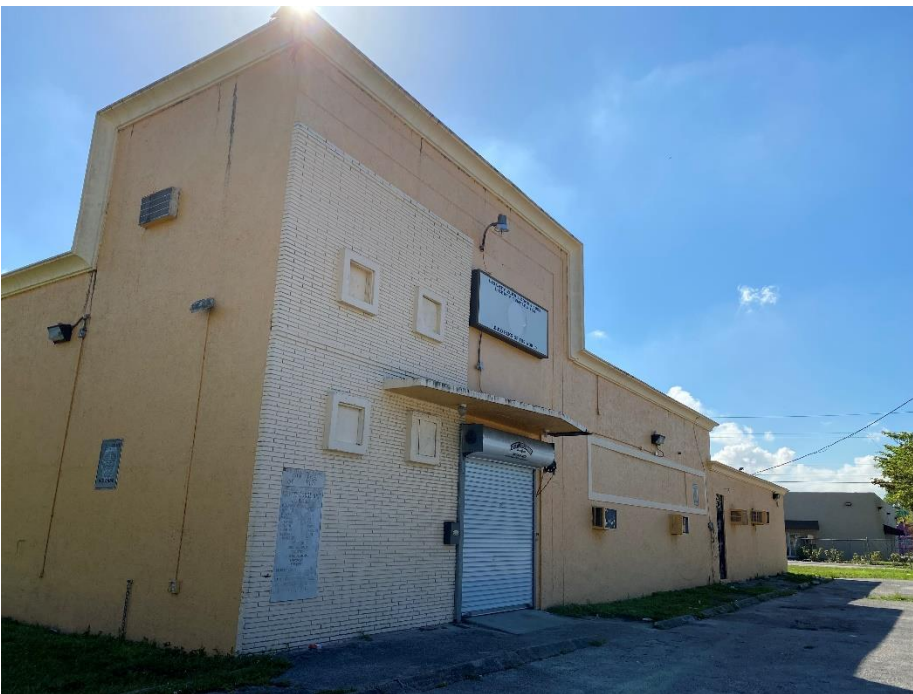
Façade/west entry of the Lodge (2021) illustrating decorative brick, four squares, fascia, entryway and signage area. The façade has been altered to enclose windows that were historically on the c.1956 building, and to enclose windows and doors on the c.1958 addition.
