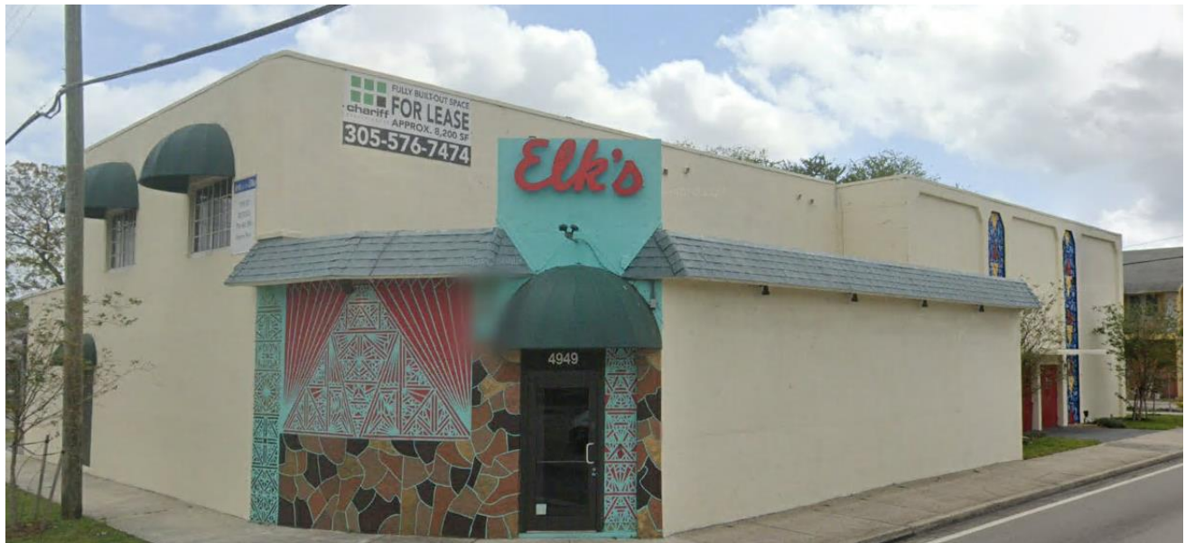
c.2020 image of the Elks Lodge at 4935-4949 NW 7 Avenue, Google Maps.
