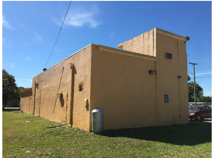
Northeast corner showing north and east elevations.
