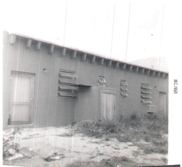
Rear of the c.1958 addition.
