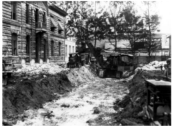
View of steam shovel being used to excavate and clear the site for the new courthouse alongside the original courthouse, visible at left, 1925. (Photo courtesy Reference Collection, Florida Memory Collection, Image No. RC19573)
