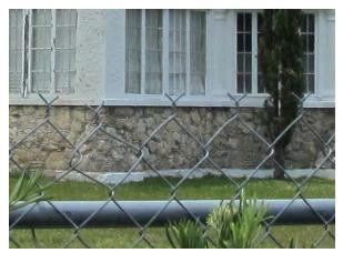
Reinforced concrete exposed footer provides support for oolitic rock walls of Masonry Vernacular home
