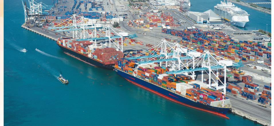
13 ship-to-shore cranes including six super Post-Panamax, the largest in the Southeastern U.S. The cranes have an outreach of 22 containers wide, stack up to nine containers high above deck, and 11 containers below deck with no height restrictions.
