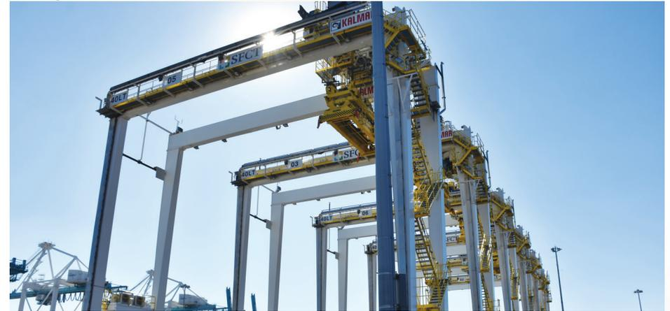
South Florida Container Terminal received 6 Electric Rubber-Tyred Gantry cranes at the beginning of 2020. Phase 1 completed in April 2021 with final Phase completion estimated to be in Q4 of 2023. RTGs greatly increase efficiencies while decreasing emissions. The electric power system removes the need for engine component maintenance, lowering downtime and reducing maintenance costs.
