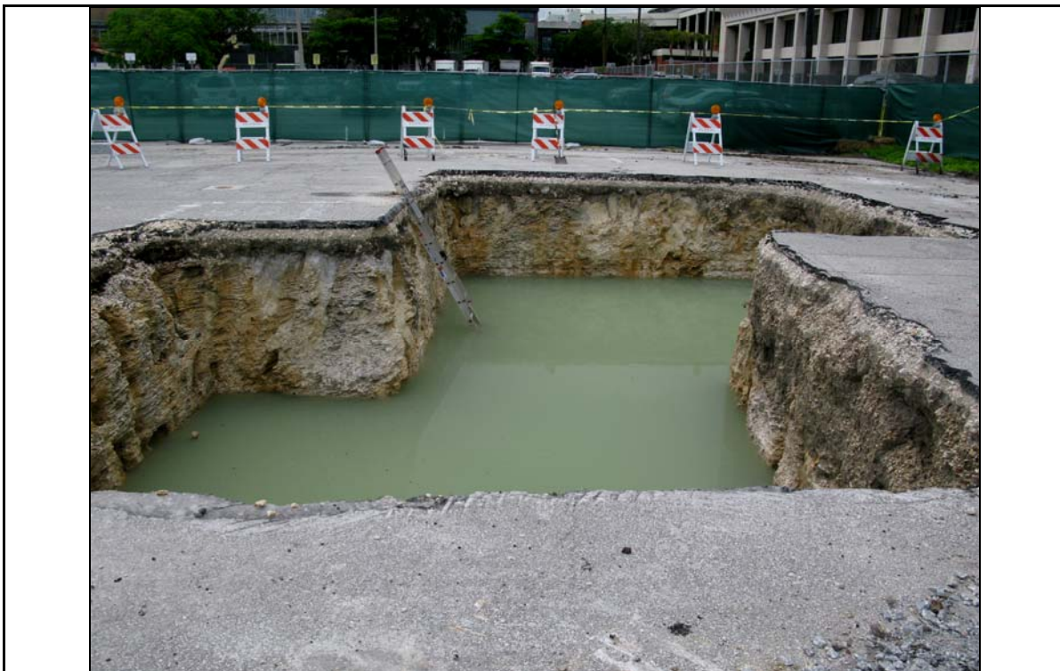
PHOTO NO. 4 DESCRIPTION: 8-Jun-09 – View of MW-17 and 18 joined excavations following FFP removal. View facing west.
