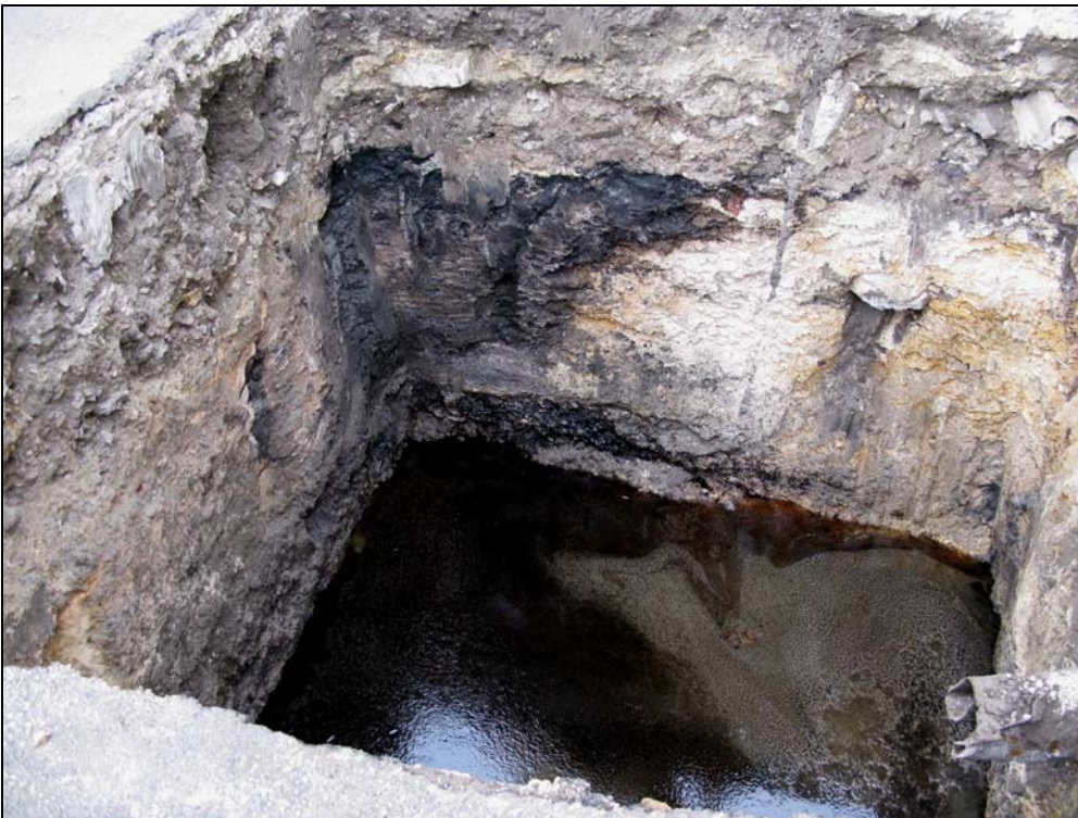
PHOTO NO. 2 DESCRIPTION: 26-May-09 – View of excavation at MW-19. Note free floating product (FFP) on groundwater table. View facing north.
