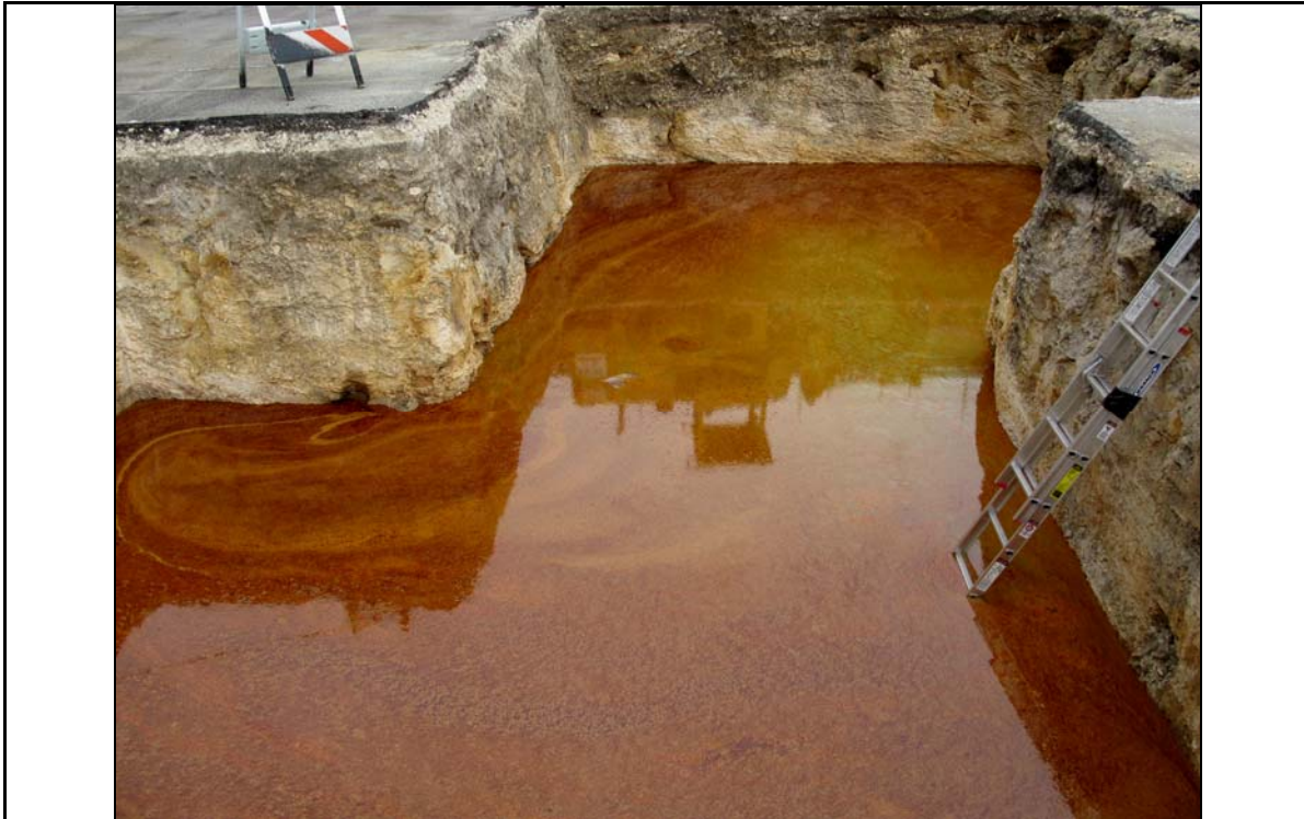
PHOTO NO. 3 DESCRIPTION: 26-May-09 – View of joined excavations MW-17 and 18. Note amber FFP. View facing east.
