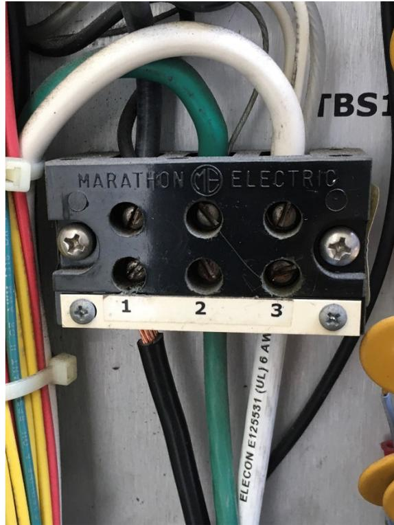
Figure 5 TBS1 Terminal Inside the Traffic Signal Cabinet
