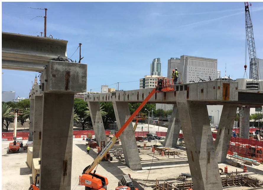
Figure 6. Viaduct construction on July 29, 2016. Photo by Phillip Pessar, posted on Flickr
