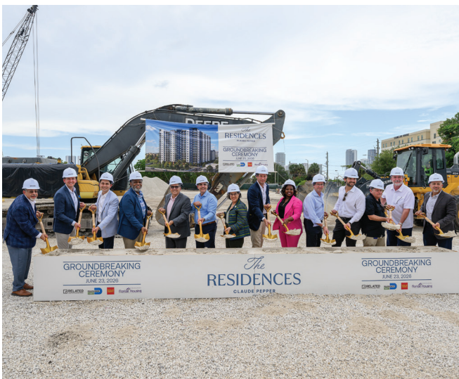
Photos By: Armando Rodriguez; Groundbreaking with local elected officials and community partners.
