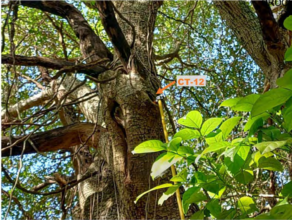
CT-12 with video camera inserted in cavity
