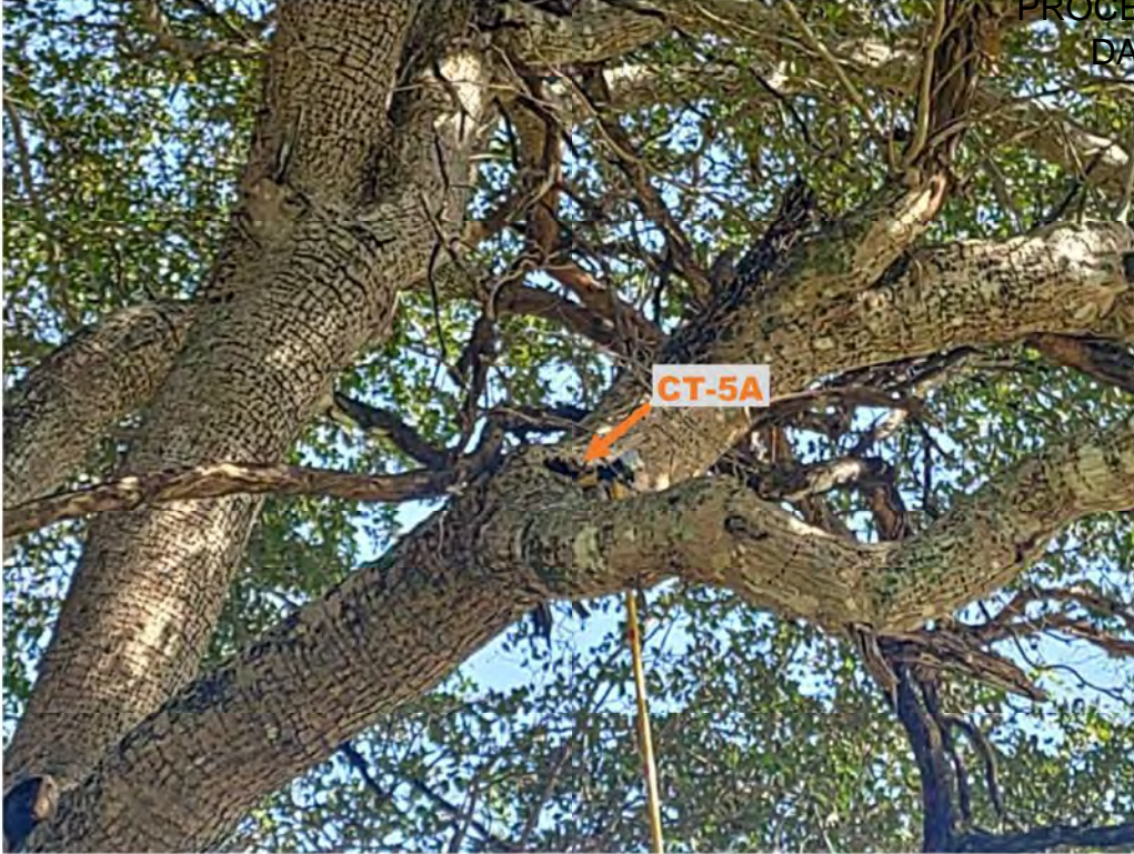
CT-5A with video camera inserted in cavity
