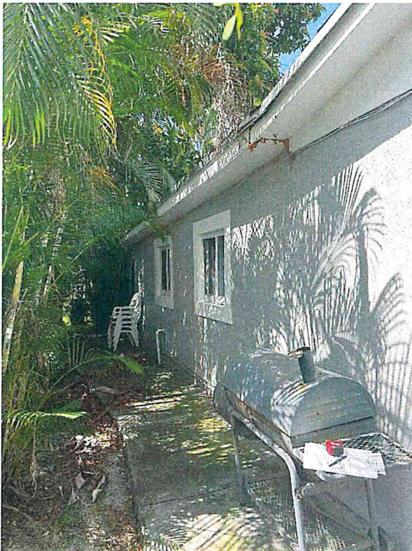
LATERAL FAÇADE, LEFT SIDE
