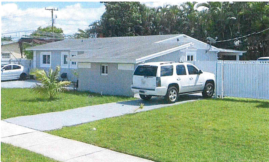
RIGHT SIDE OF FRONTAL FAÇADE
