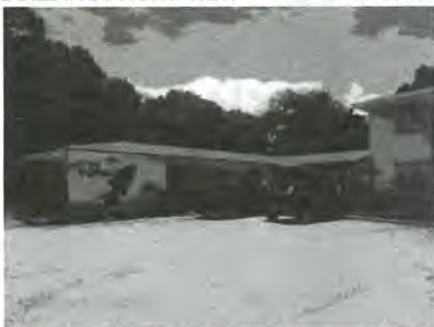
BUILDING FRONT VIEW
