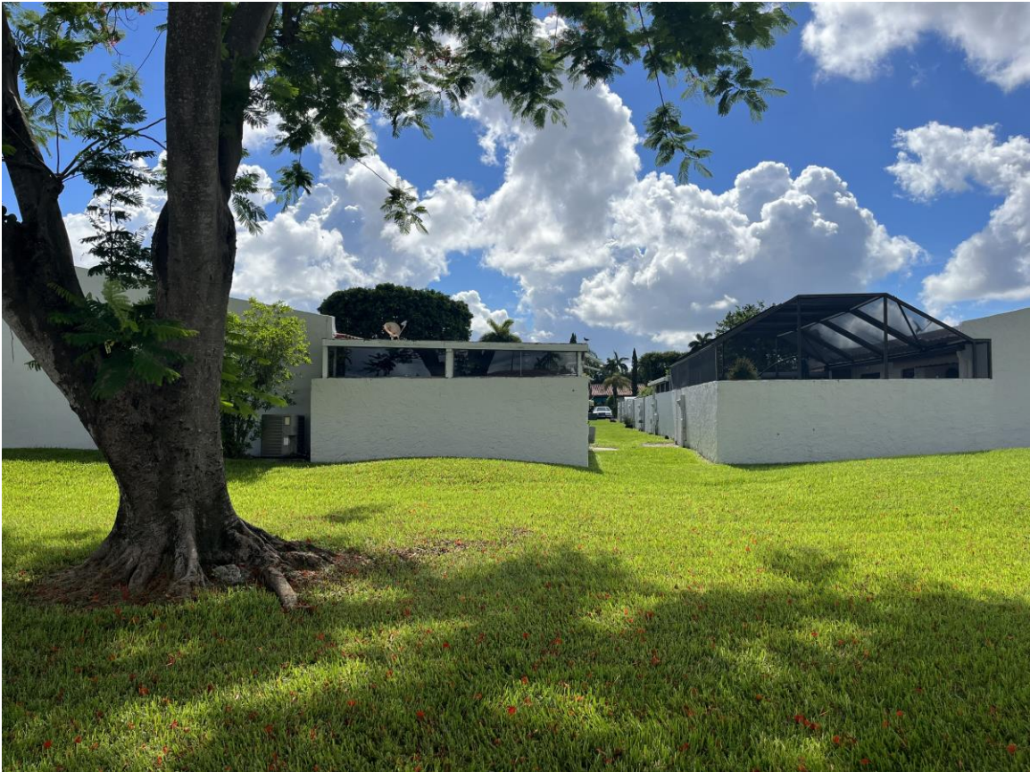
SIDE OF PROPERTY
