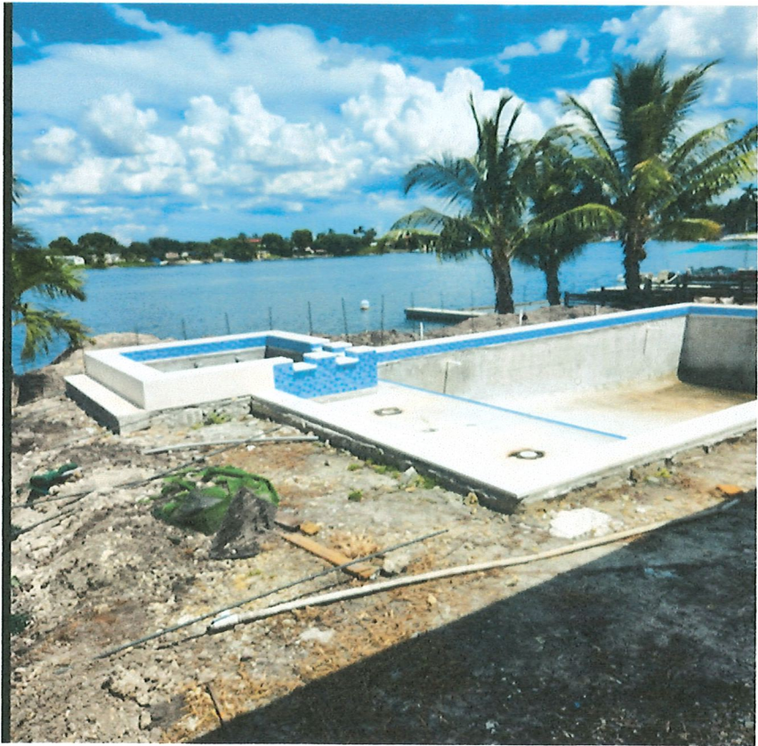
LATEST VIEW OF SUBJECT PROPERTY
