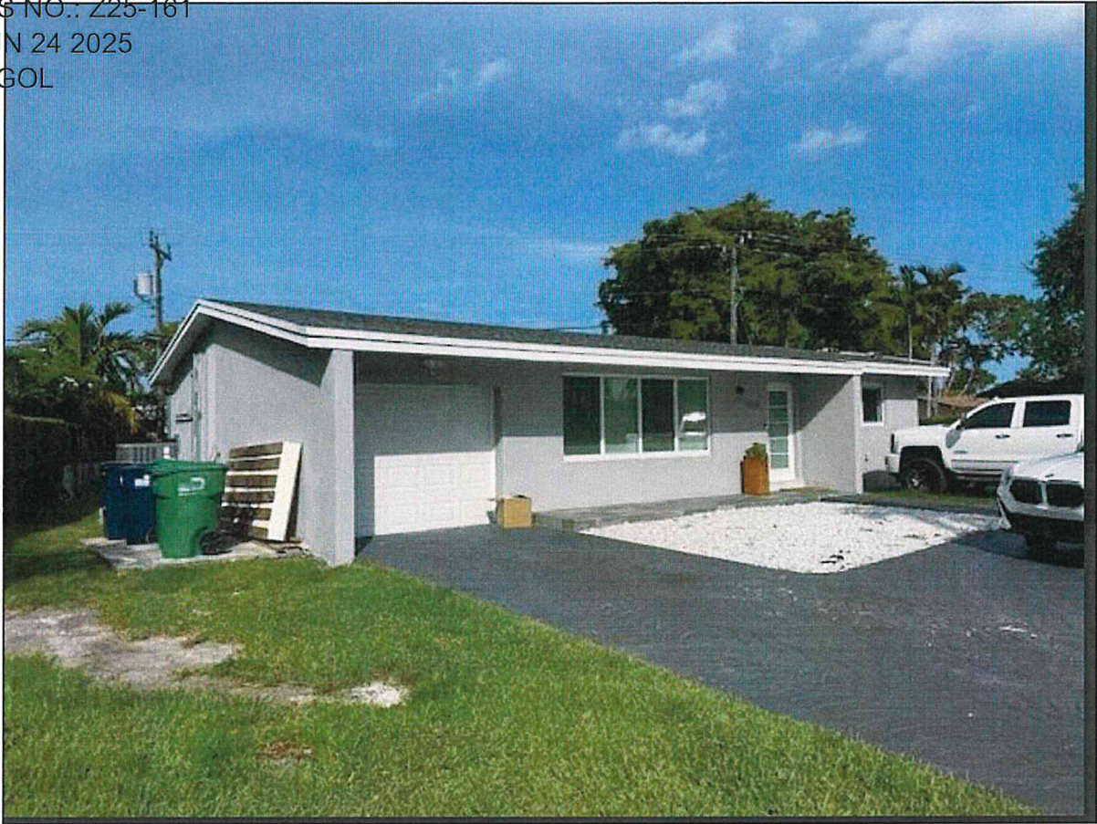
FRONT INTERIOR SIDE VIEW FACING EAST
