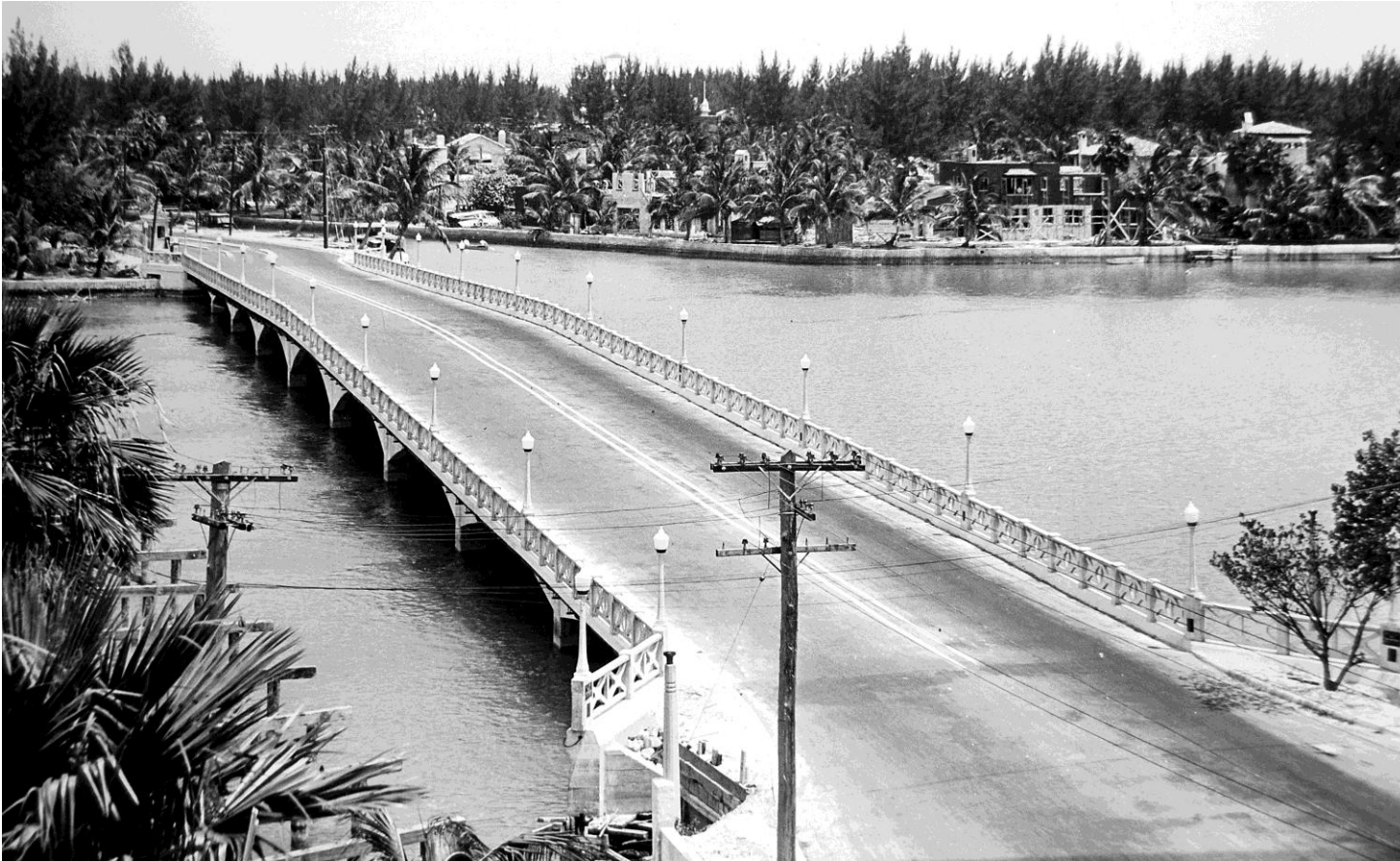
Aerial View of Bridge 12 of the Venetian Causeway c. 1930.
