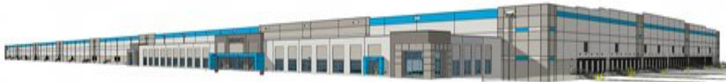
HOMESTEAD FULFILLMENT CENTER 1000 SW 10TH AVENUE, MIAMI, FL 33135
