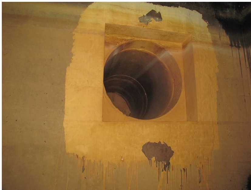
Photo #11. Overflow valve on the west wall.
