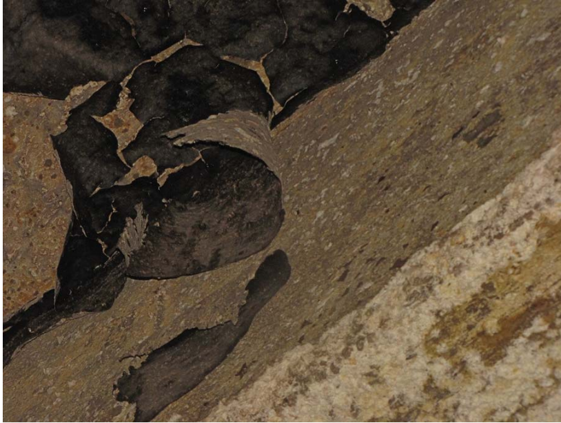
Photo #6. Detail of paint film peeling off the concrete surface.
