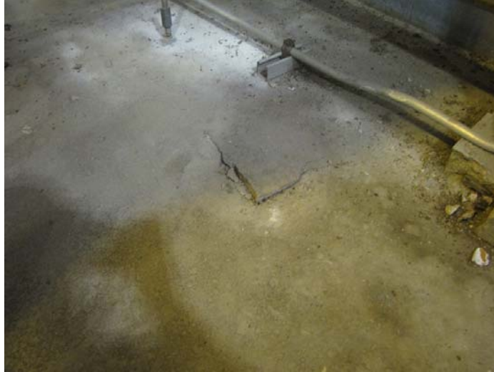
Photo #2. Upper side of slab. Minor concrete deterioration
