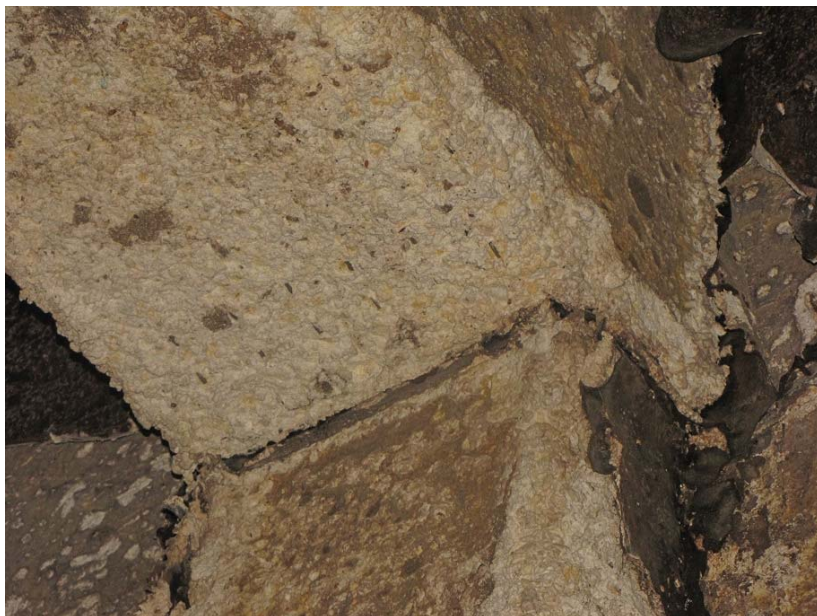
Photos #7. Detail of efflorescence.
