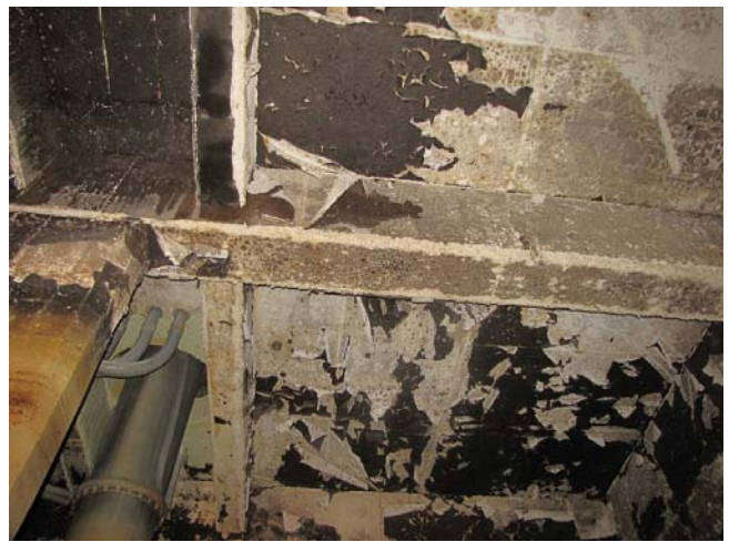
Photos #4 and #5. Paint film peeling off and efflorescence.
