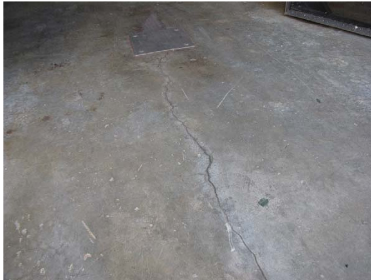
Photo #1. Upper side of slab. Minor d-crack
