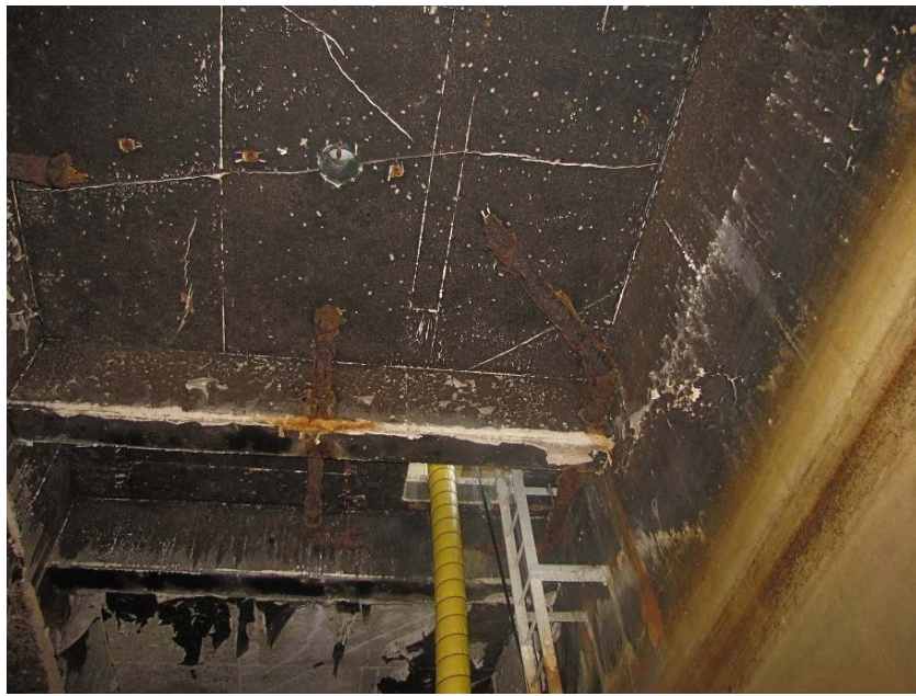
Photo #8. Some minor d-cracks on the roof slab
