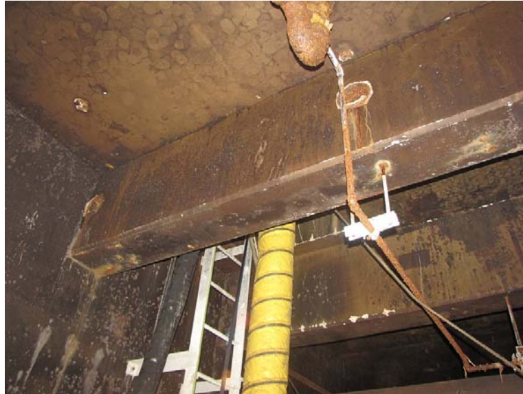
Photo #3. Some minor concrete spalling and cracking
