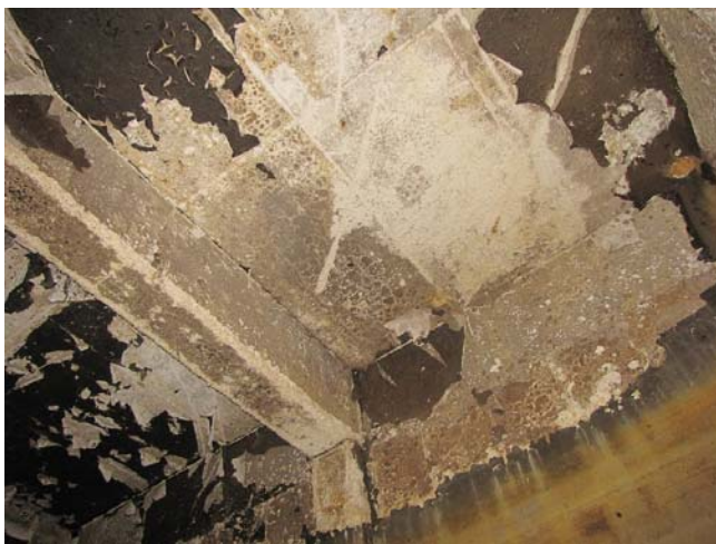
Photos #4 and #5. Paint film peeling off and efflorescence.
