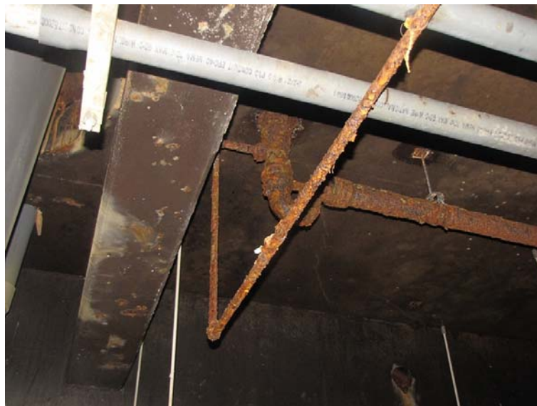
Photo #11. Corroded drainage system
