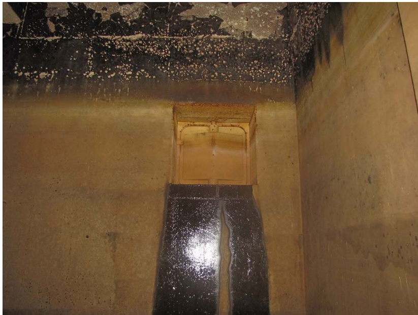
Photo #10. Butterfly valve on the east wall connecting to wet well #3.
