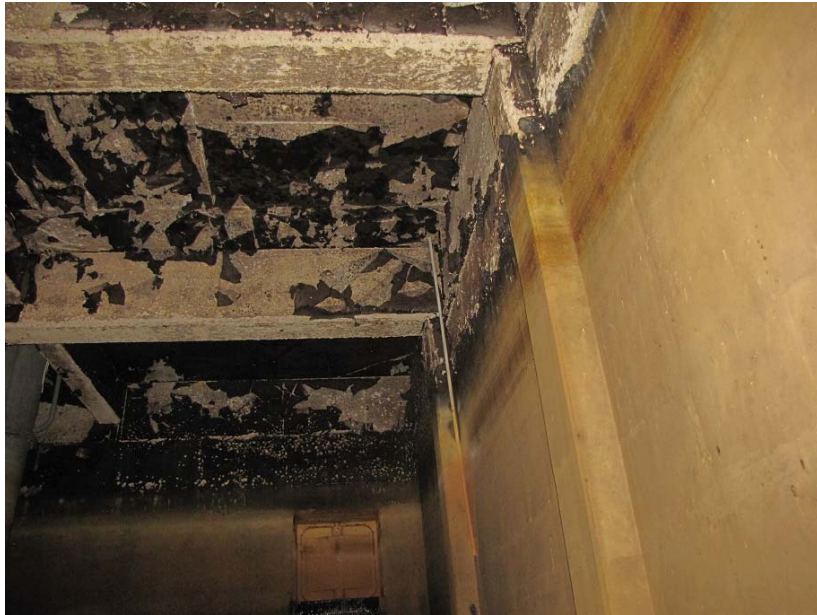
Photo #3. South-eastern wall and ceiling. Efflorescence on the dry/upper areas.
