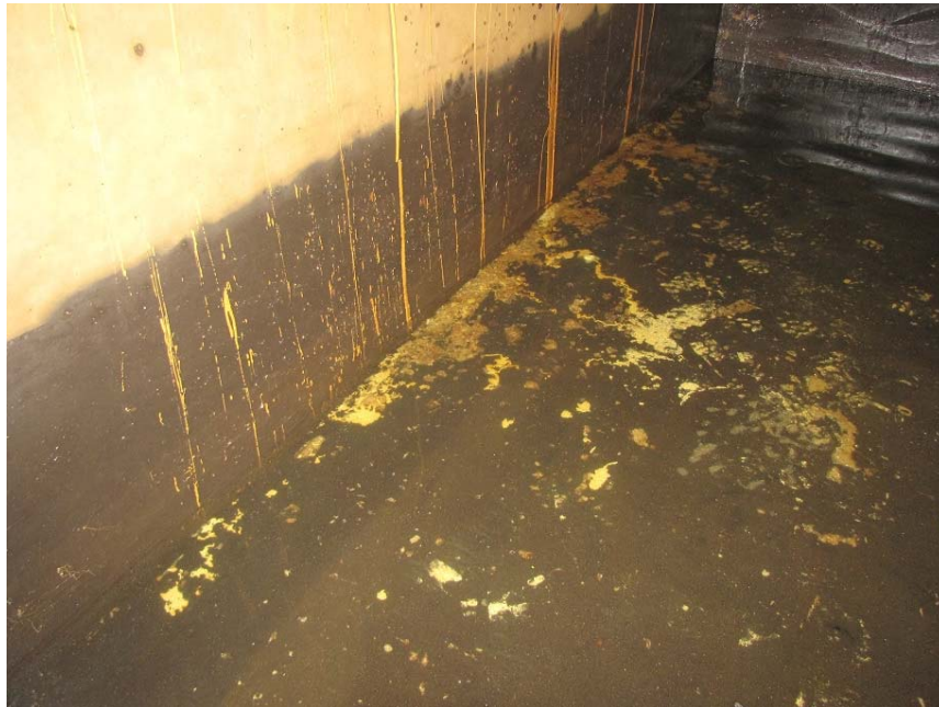
Photo #9. Spalling/scaling on floor concrete.
