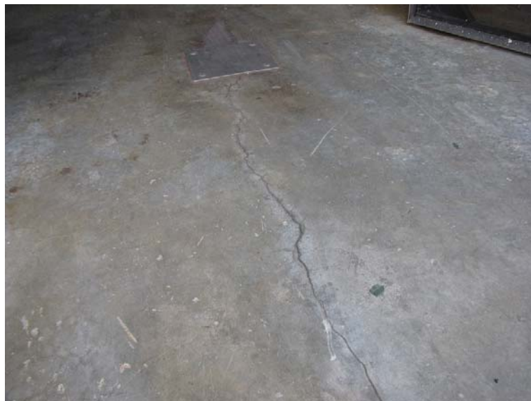
Photo #1. Upper side of slab. Minor d-crack
