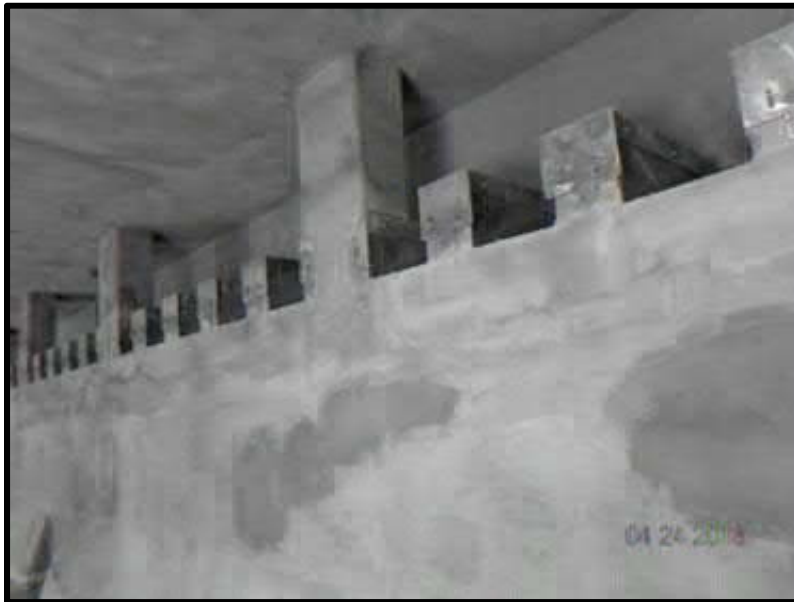
Photo 3: Resurfaced weir wall
