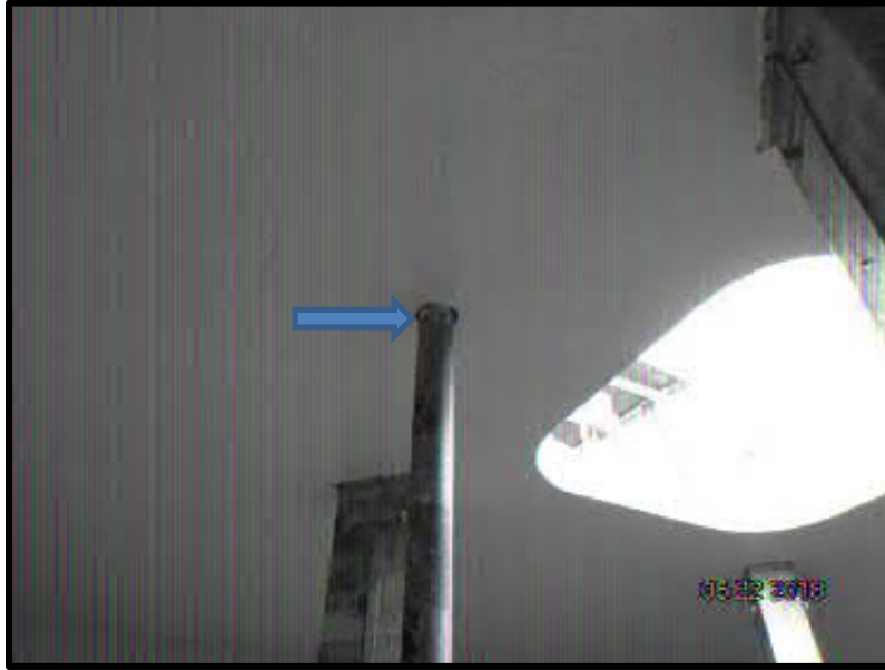
Photo 9: Roof deck pipe inserts - Before
