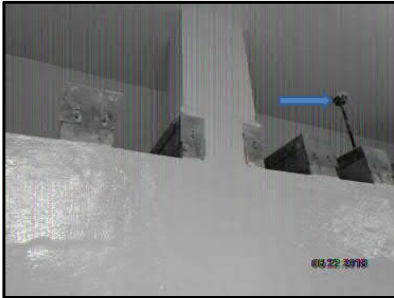
Photo 10: Valve roof deck insert - Before
