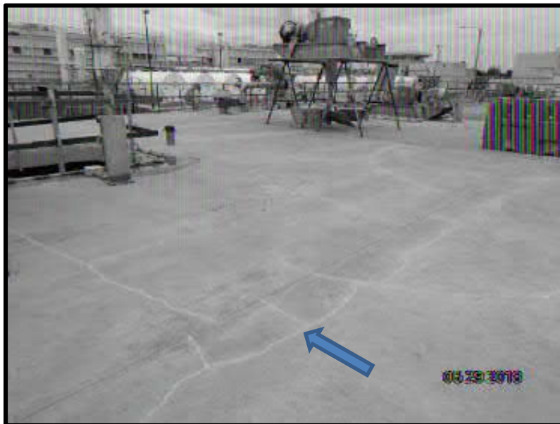
Photo 11A: Roof deck exterior cracks - After
