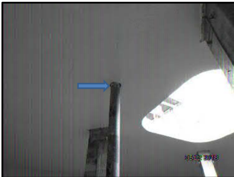
Photo 9: Roof deck pipe inserts
