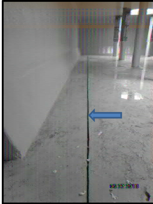
Photo 5: Floor slab expansion joint – Area No. 2 - Before
