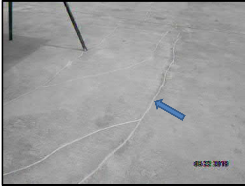
Photo 11: Roof deck exterior cracks - Before
