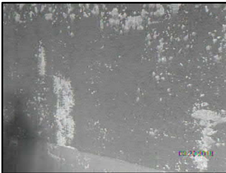
Photo 6: Surface prior abrasive blasting
