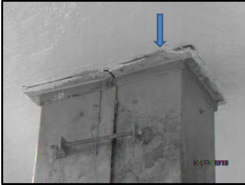
Photo 3: Concrete column corner guard top edge - Before
