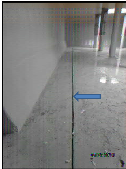
Photo 5: Floor slab expansion joint – Area No. 2
