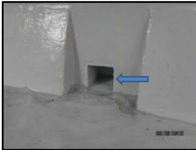
Photo 12A: Weir wall 1ft x 1ft opening – Area No. 6 – After
