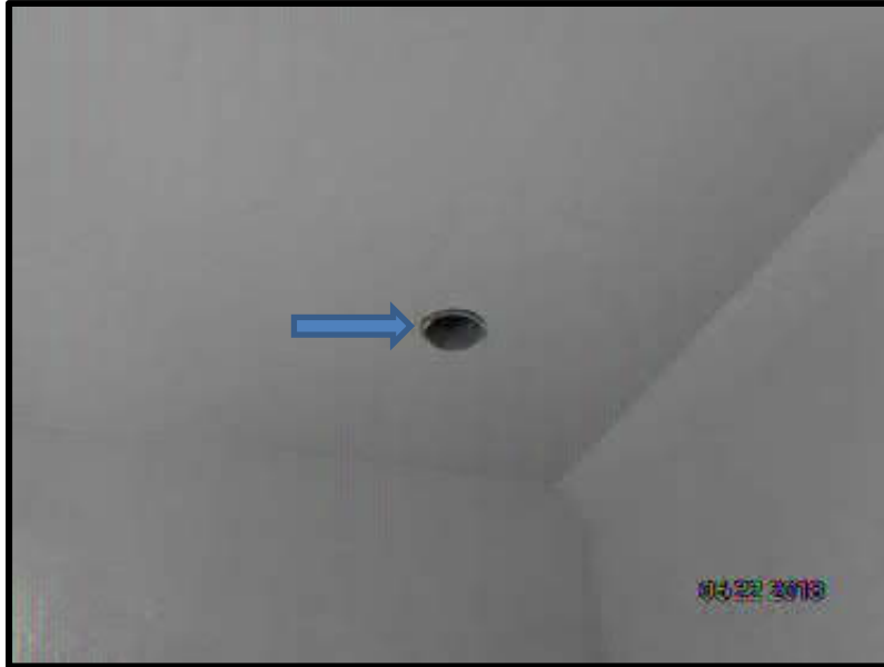
Photo 8: Roof deck pipe inserts
