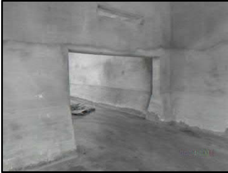
Photo 2: Resurfaced baffle wall
