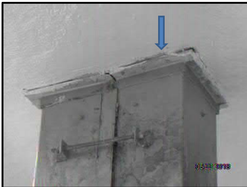
Photo 3: Concrete column corner guard top edge
