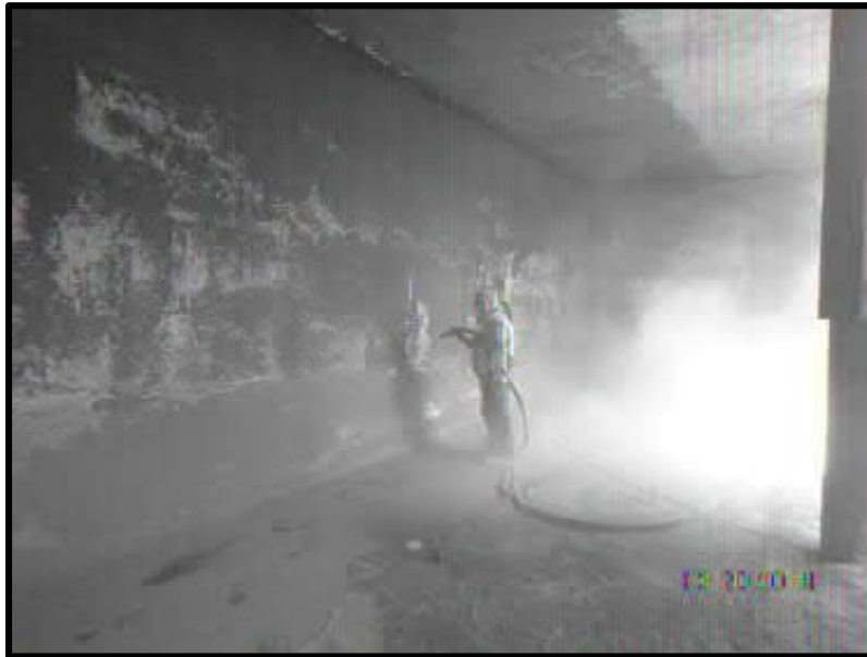
Photo 7: Abrasive blasting procedure
