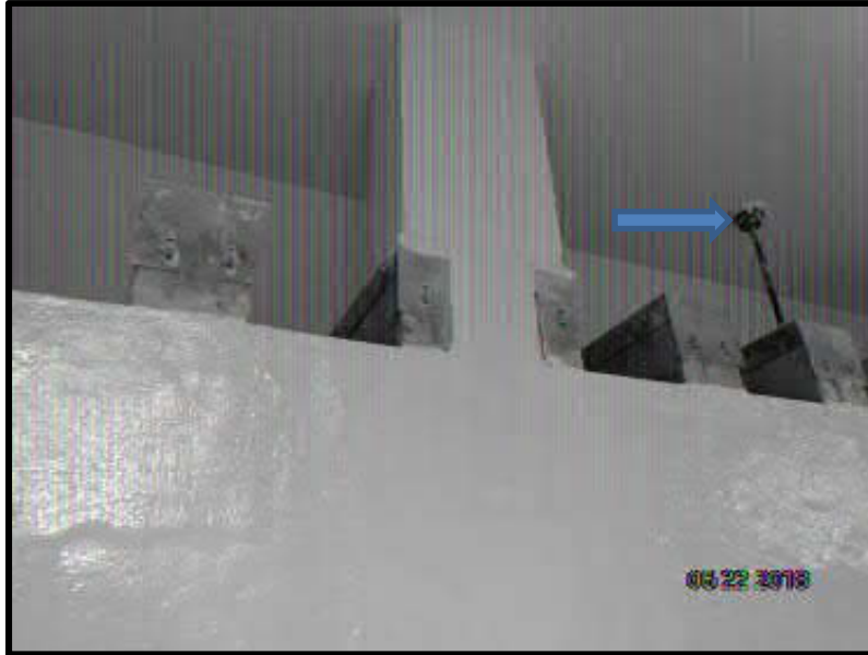
Photo 10: Valve roof deck insert
