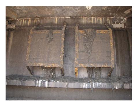
Photo #21. Influent valve protective baffles. No sign of leakage.
