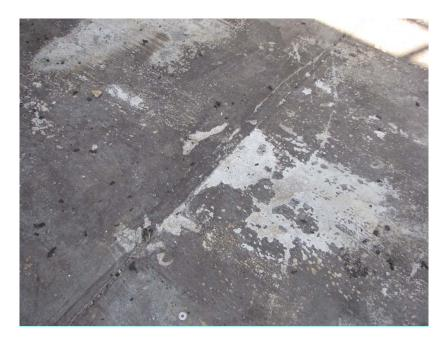
Photo #12. Transversal crack along the W-E construction joint. Central lane.
