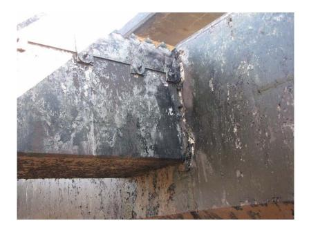
Photo #16. Gutter-trough connection. See leakage on the slip joint.
