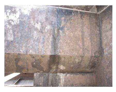
Photo #17. Leakage on a trough expansion joint.
