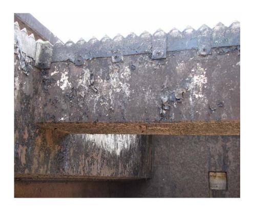
Photo #15. Efflorescence and concrete deterioration on the effluent gutters.
