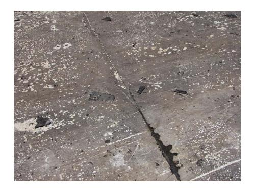
Photo #13. Transversal crack along the W-E construction joint. Eastern lane.
