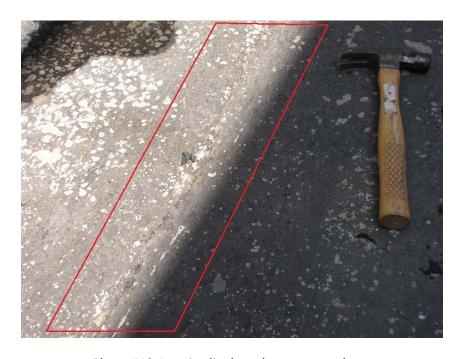
Photo #10. Longitudinal crack on western lane.
