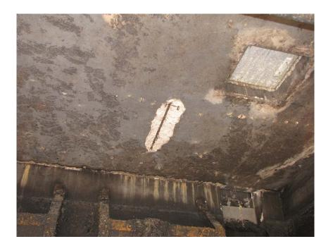
Photo #7. Exposed reinforcement steel. North underslab of Eastern Lane
