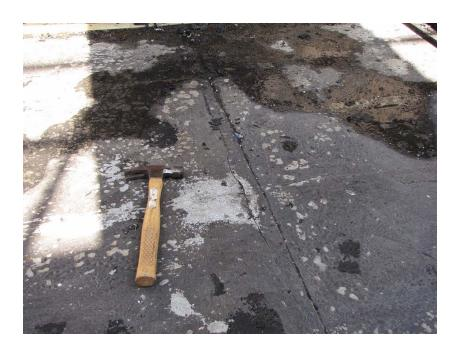
Photo #11. Transversal construction/contraction joint and crack. Western lane.
