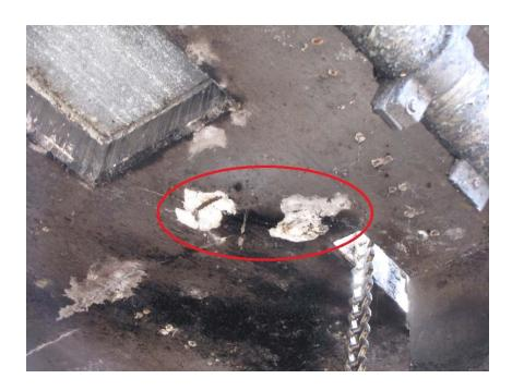
Photo #6. Exposed reinforcement steel. North underslab of Western Lane.
