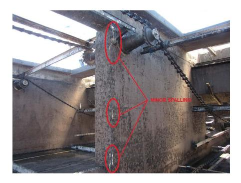
Photo #2. Concrete spalling on intermediate central wall
