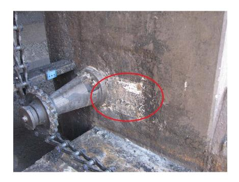
Photo #3. Blistering and concrete spalling on intermediate northern wall
