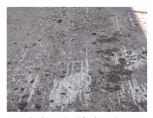
Photo #9. Loose coating on the floor of the central lane. Concrete scratches on the direction of the moving sludge conveyor.
