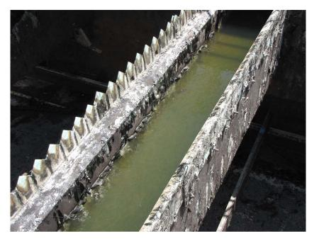
Photo #18. Effluent Gutter weirs.
