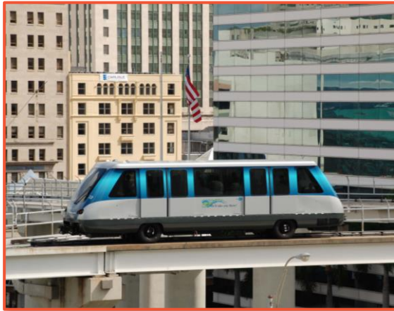
Automated Guideway Transit
