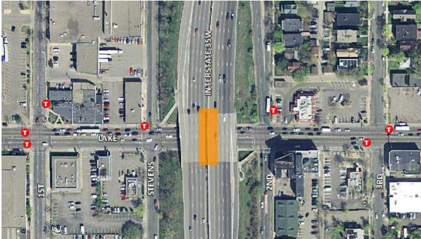
I-35 W & Lake Street Street Station Aerial
