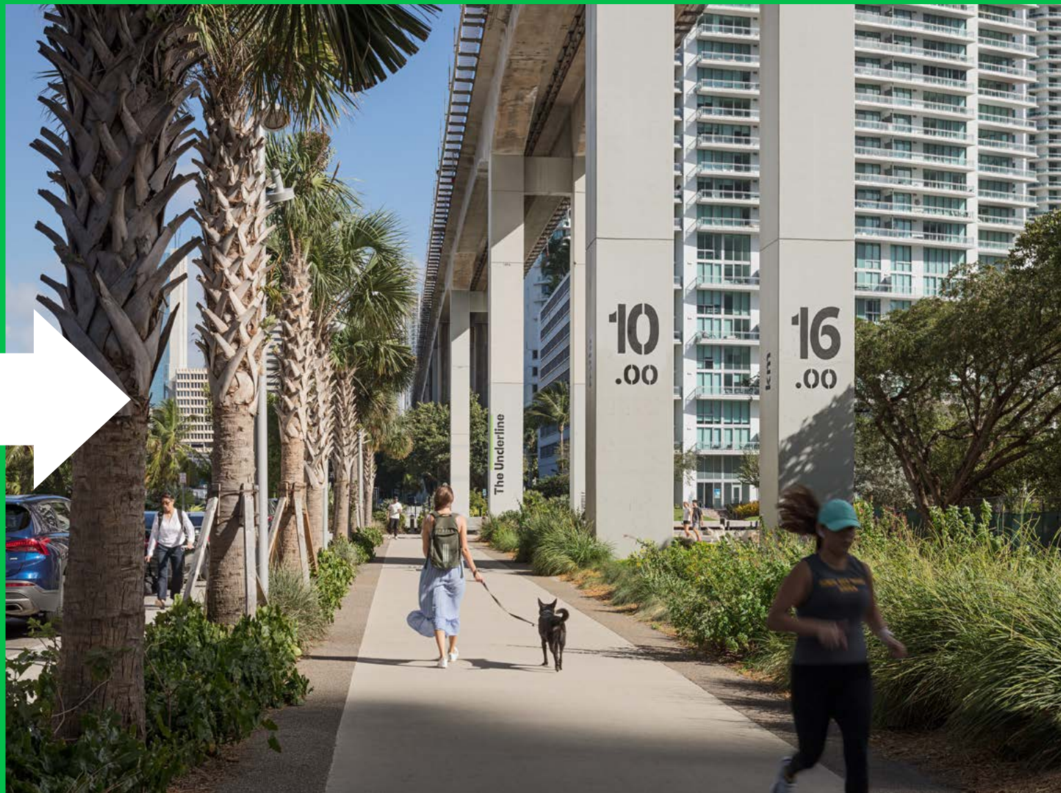
Phase 1 Brickell Backyard- After
