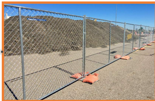
Chain Link Fence at Intersections
