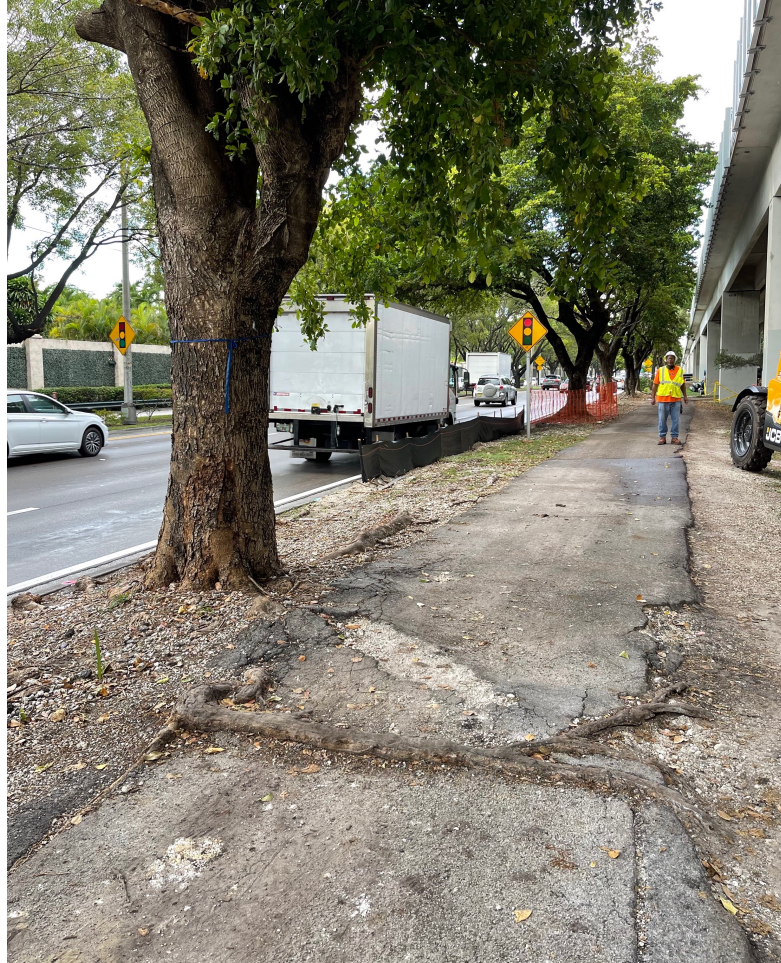
Roots cracking path
