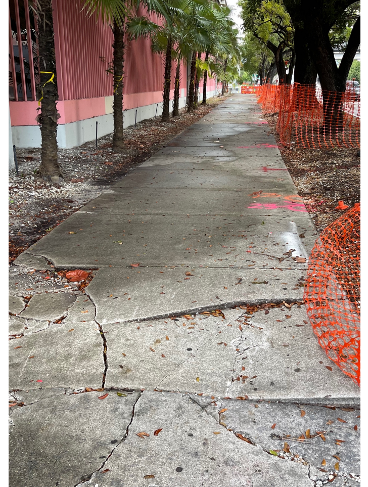
Roots cracking path
