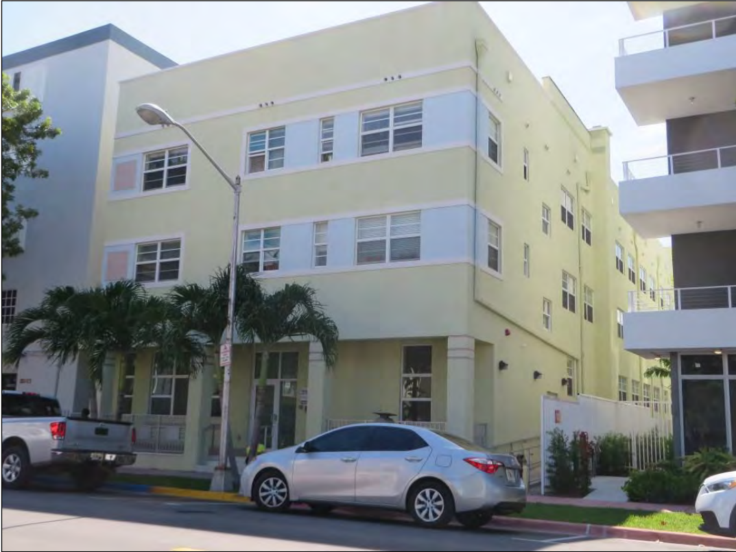
Figure 22. Resource 8DA11652, facing southwest within the Beach Corridor APE.
