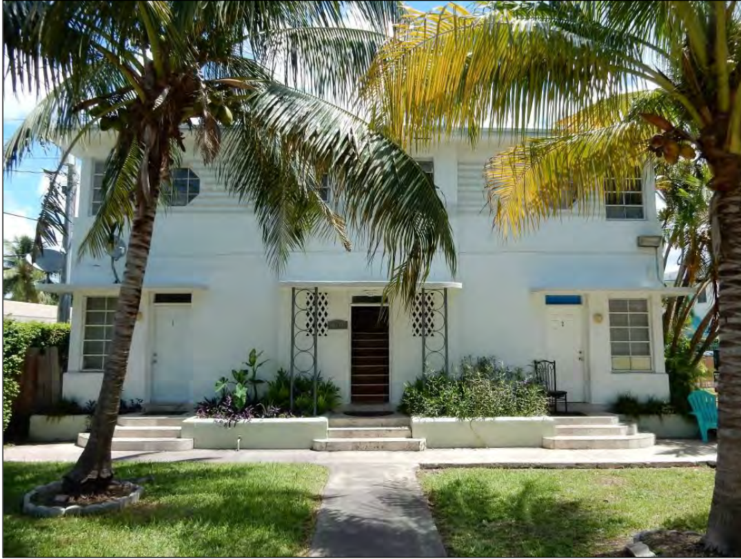
Figure 26. Resource 8DA18057, facing east within the Beach Corridor APE.
