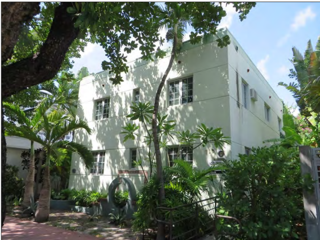
Figure 47. Resource 8DA18085, facing southwest within the Beach Corridor APE.
