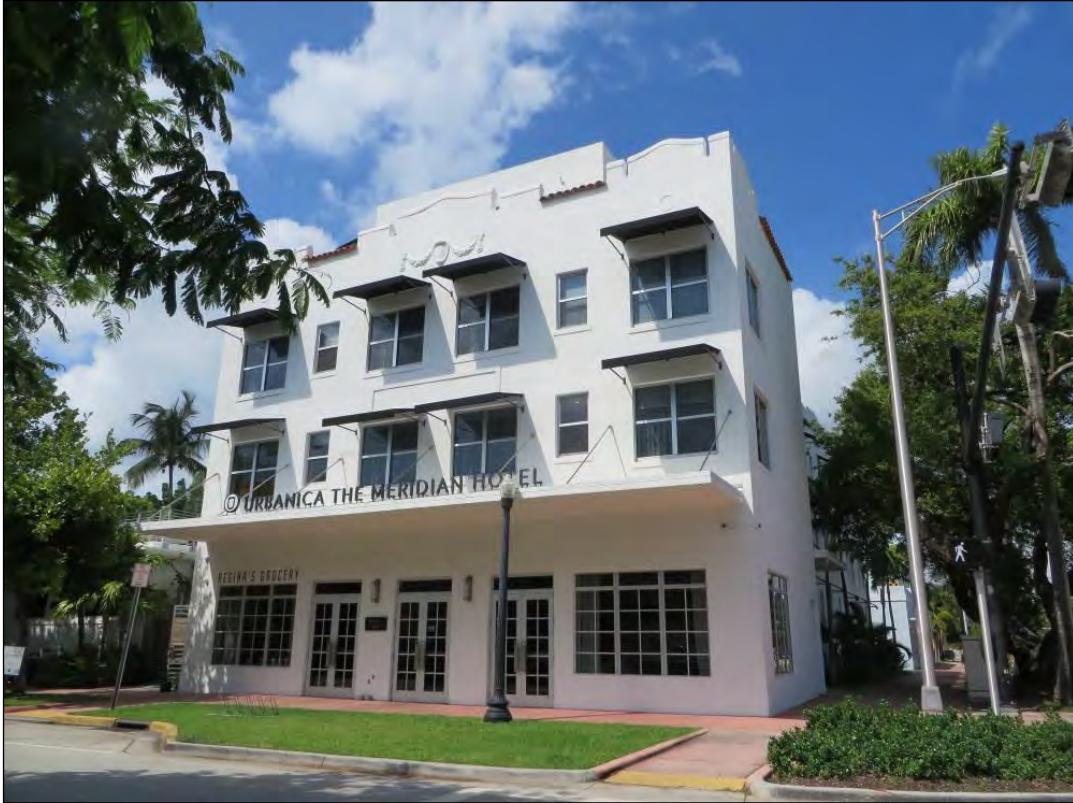
Figure 48. Resource 8DA18086, facing southwest within the Beach Corridor APE.
