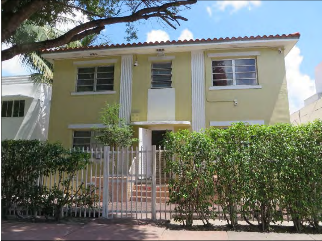
Figure 52. Resource 8DA18091, facing east within the Beach Corridor APE.
