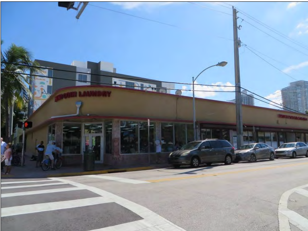
Figure 51. Resource 8DA18090, facing southwest within the Beach Corridor APE.
