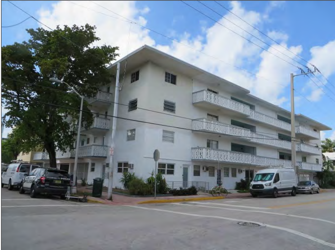
Figure 41. Resource 8DA18076, facing southwest within the Beach Corridor APE.
