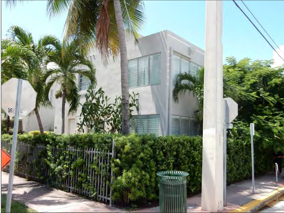
Figure 28. Resource 8DA18059, facing southwest within the Beach Corridor APE.
