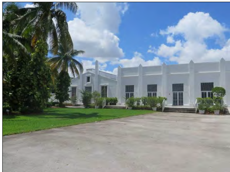
Figure 10. Resource 8DA10520, facing southwest within the Beach Corridor APE.
