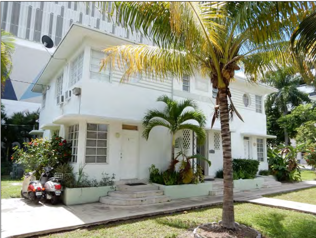
Figure 25. Resource 8DA18056, facing southwest within the Beach Corridor APE.
