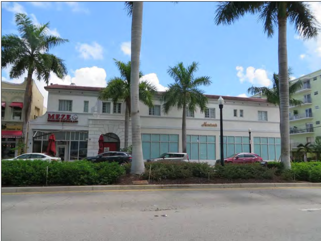
Figure 61. Resource 8DA18112, facing east within the Beach Corridor APE.
