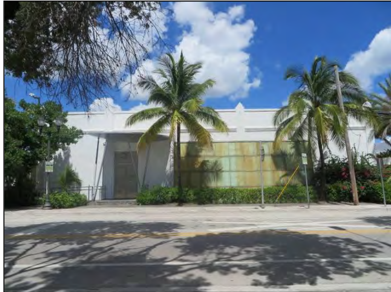
Figure 12. Resource 8DA10858, facing north within the Beach Corridor APE.
