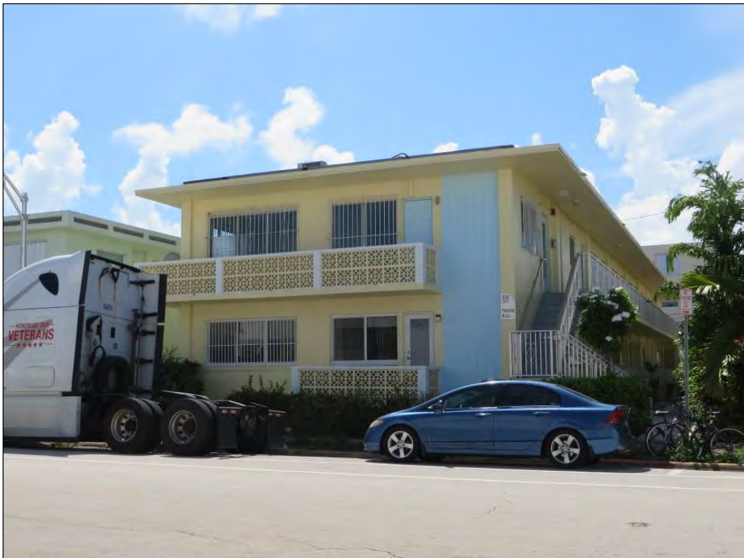
Figure 57. Resource 8DA18102, facing southwest within the Beach Corridor APE.
