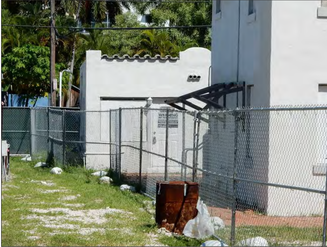
Figure 34. Resource 8DA18068, facing east within the Beach Corridor APE.
