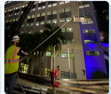
Delivery of track switch main pivot beam
