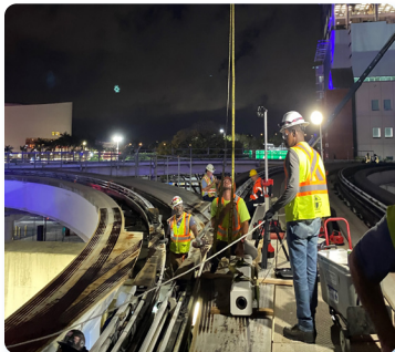
Track switch replacement
