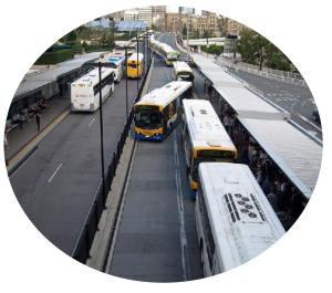
lane and dedicate it to exclusive BRT infrastructure, especially with limited right of ways. Another design alternative is installing a pull-by in front of the BRT station where a local bus can move out of the way of an express bus if the driver sees one coming.
