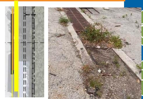
Demolition and removal of 670 LF of trench drains (out of service)
