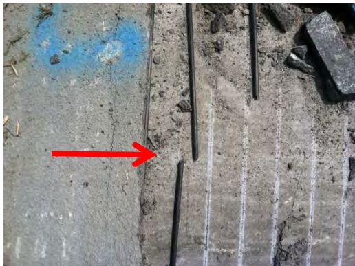
Figure 3.5 Brittle wire fracture observed following the removal of the mortar coating.
