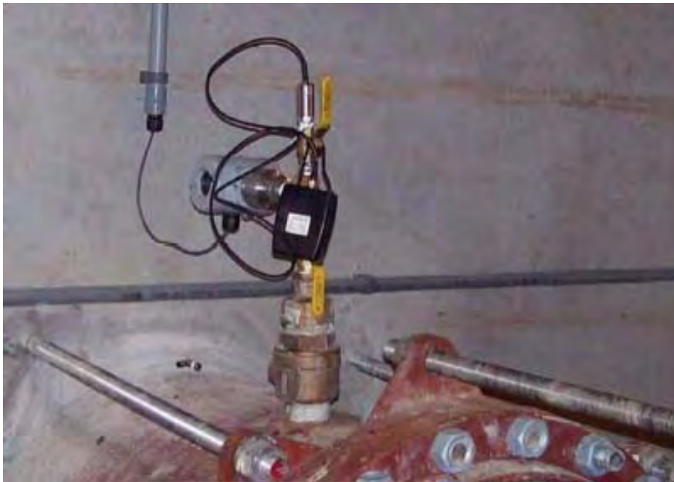
Figure 6-1 - Example Pressure Logger Installation
