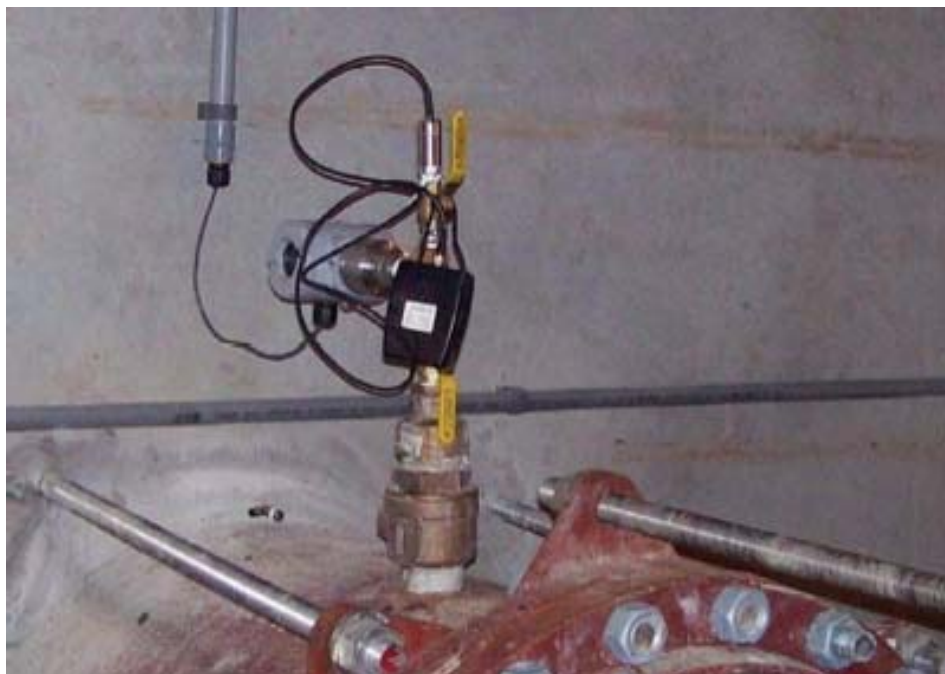
Figure 6-1 Example Pressure Logger Installation
