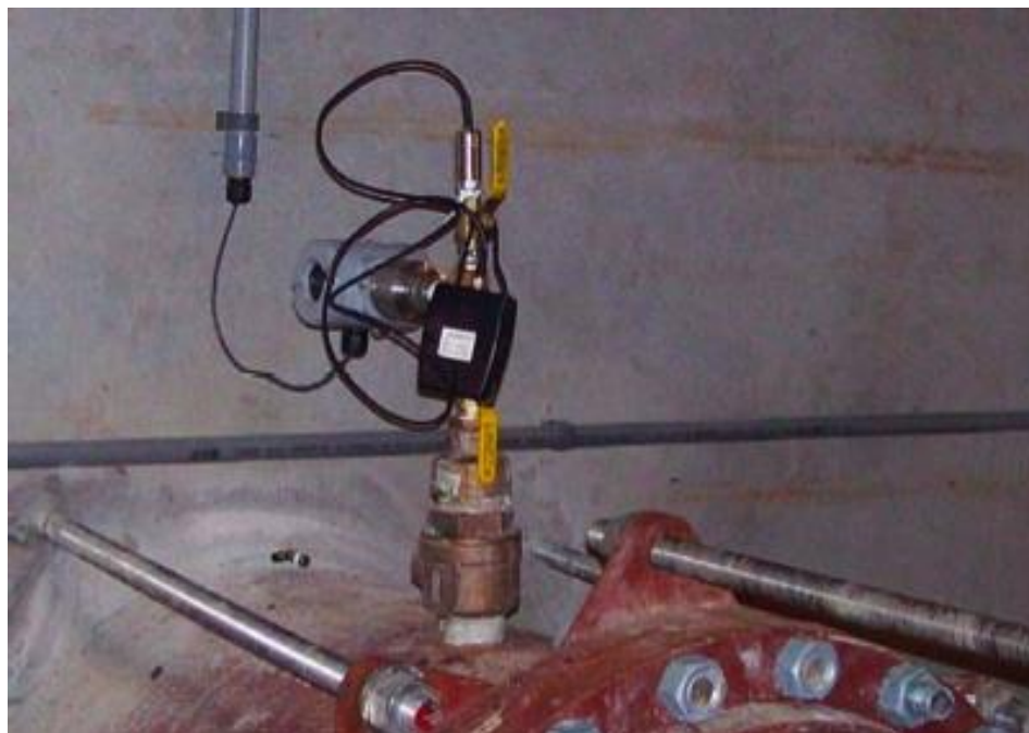
Figure 6-1 Example Pressure Logger Installation
