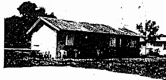
Figure 98. Homestead Housing (Before)
