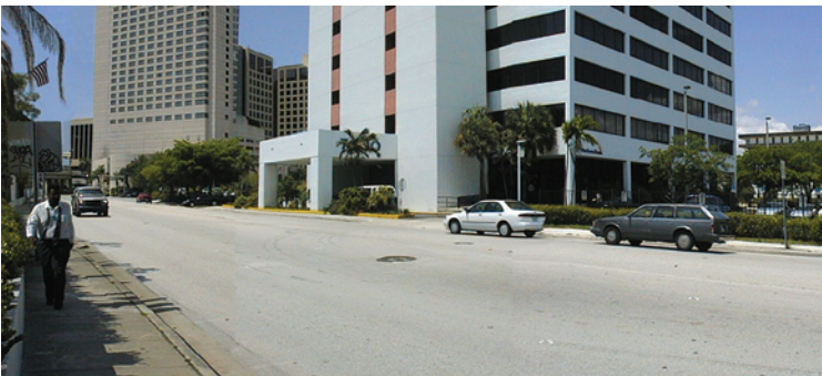
Above: Before and After of Dadeland Boulevard
