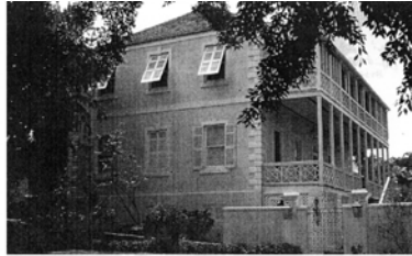
Masonry construction, Bahama shutters
