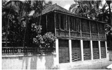
Masonry and wood construction, louvers
